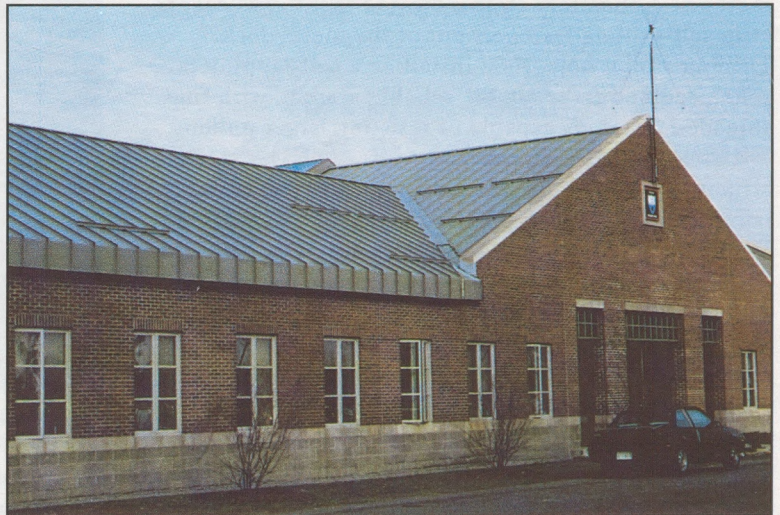
Figure 8: Array of six aluminum angle snow guards used to protect a valley and, to the left, a single guard to study "worst case" loading.
