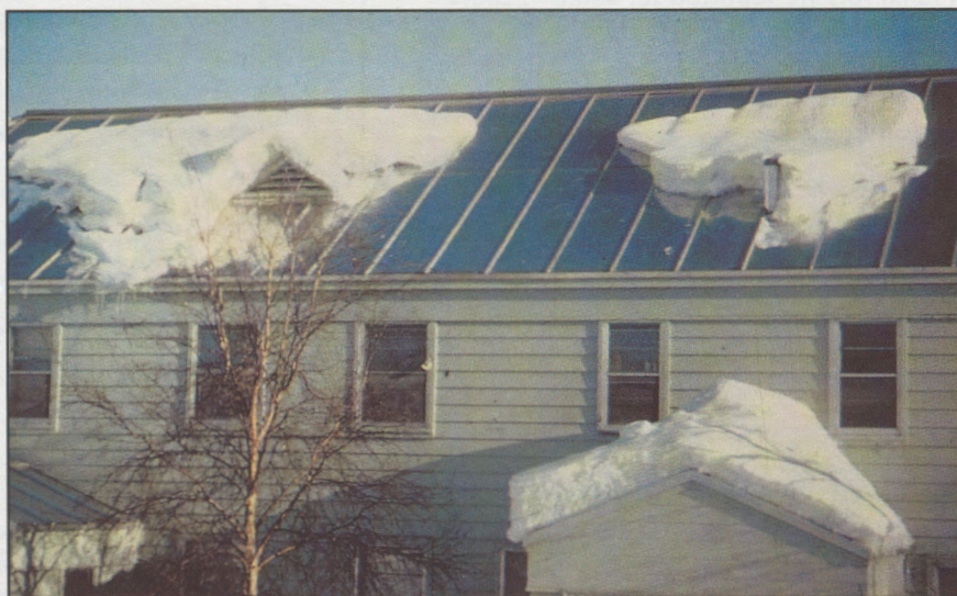
Figure 5: A small object such as a plumbing vent can hold back a large wedge of snow.
