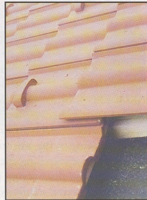
These tiles have affixed concrete snow stops. Note the vented system between deck and tile, at right.
