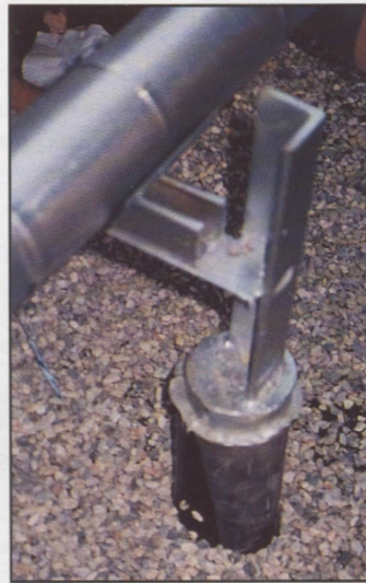
Angle iron support flashed with a lead roof jack.
