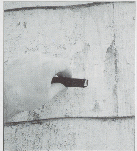
This penthouse siding is highly friable. Roofing work often encounters such conditions. These areas must be identified and addressed in the specifications.
