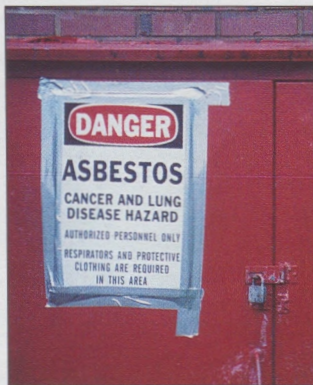
Proper posting of the jobsite and disposal of regulated asbestos are just two of many requirements on a project with regulated asbestos.
