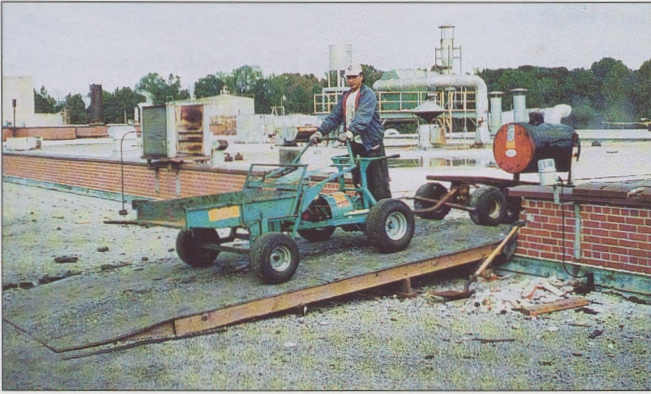
Powered carts hauling luggers and moving hundreds of pounds of material will always affect the deck and anything attached to the deck's underside.
