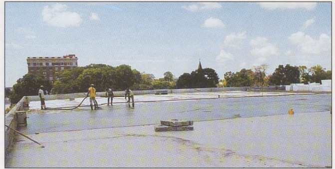
(Left) The cellular insulating concrete pour is in progress, with filler boards being set in the slurry. (Above) 2" to 3" of cellular concrete are being poured over the stepped insulation boards.
