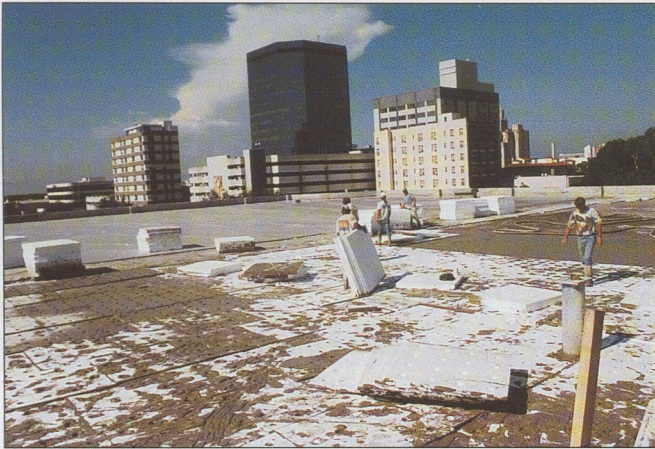
(Left) The cellular insulating concrete pour is in progress, with filler boards being set in the slurry. (Above) 2" to 3" of cellular concrete are being poured over the stepped insulation boards.
