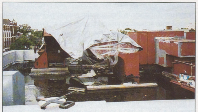
(Left) The rusting supports for the old cooling tower were left on the roof. (Right) Unused HVAC equipment was covered with tarps because leaking occurred through it.
