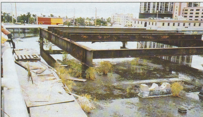
(Left) The rusting supports for the old cooling tower were left on the roof. (Right) Unused HVAC equipment was covered with tarps because leaking occurred through it.
