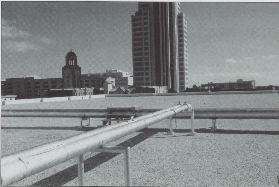
The new, completed roof.
