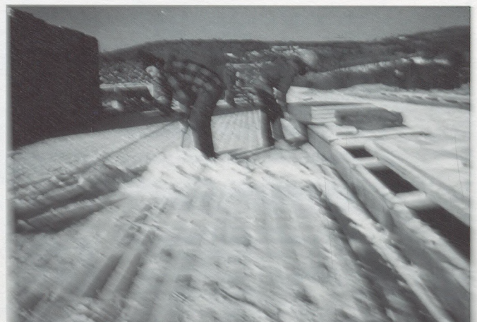
Photo 2: Snow removal from a deck in preparation for roofing.
