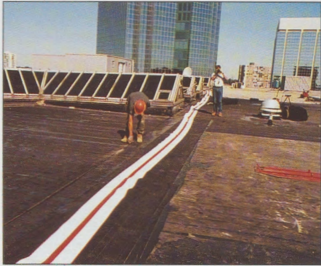
Fig. 5: The building expansion joint being prepared for roof expansion joint installation.
