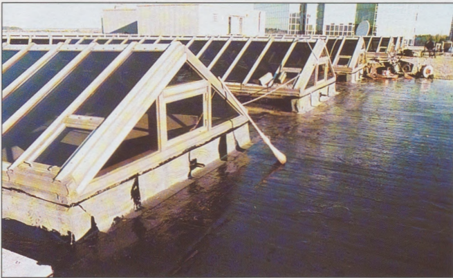
Fig. 9: The completed installation of the flat roof expansion joint. Note the vertical flashings.
