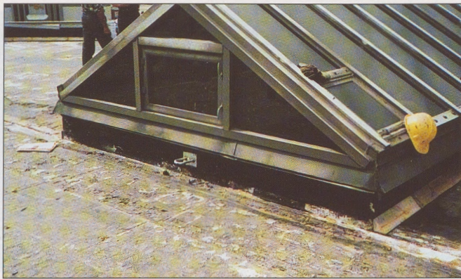
Fig.: 1 View of roof with skylights and expansion joint.
