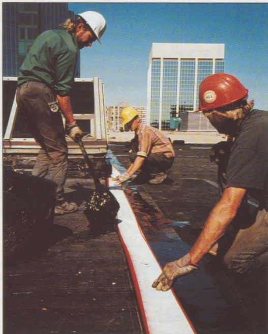
(Left): Fig 6: The roof expansion joint being installed in a flood coat of asphalt.
