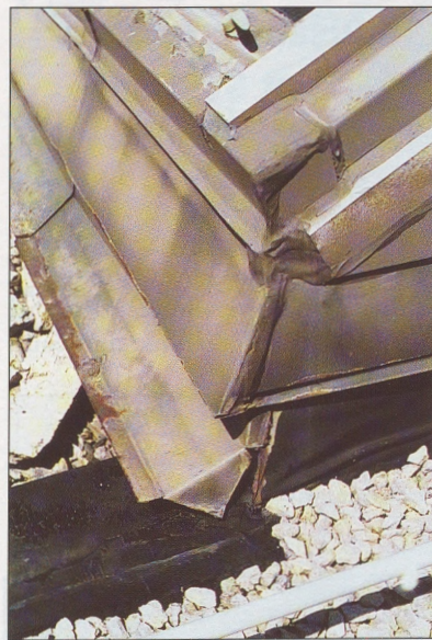
Fig.: 3 Close up of existing expansion joint at skylight curb corner.
