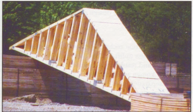
Figure 2: Bundle of pitched gable and trusses. Having only vertical web elements, these are to be supported along the entire length of the end walls.
