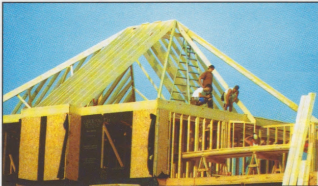
Figure 1: Built-in-place (stick-built) framing.
