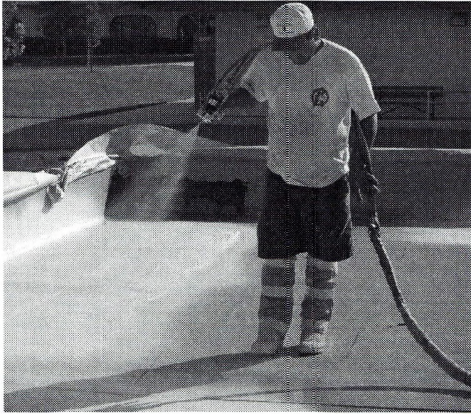
Application of SPF from trailer-mounted spray rig.
