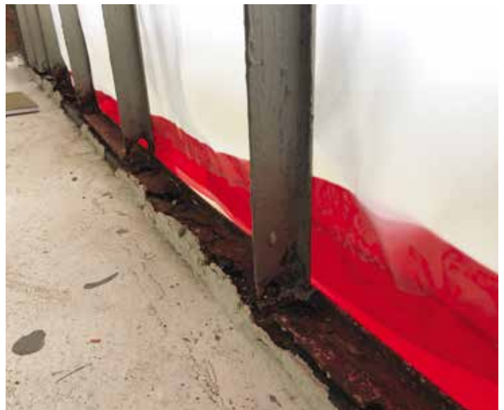
Figure 2a. Coating and glazing putty conceal corrosion of steel mullions. Figure 2b. Coating removal reveals extensive corrosion of steel mullions.
