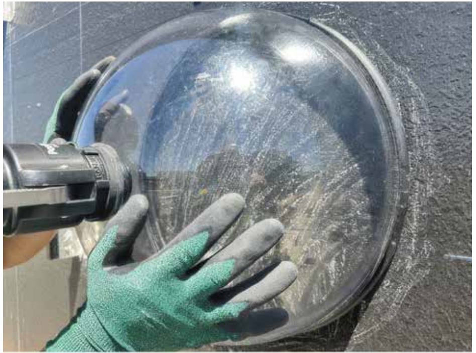
Figure 4. Testing process per ASTM E1186, Standard Practices for Air Leakage Site Detection in Building Envelopes and Air Barrier Systems. No bubble formation was observed.
