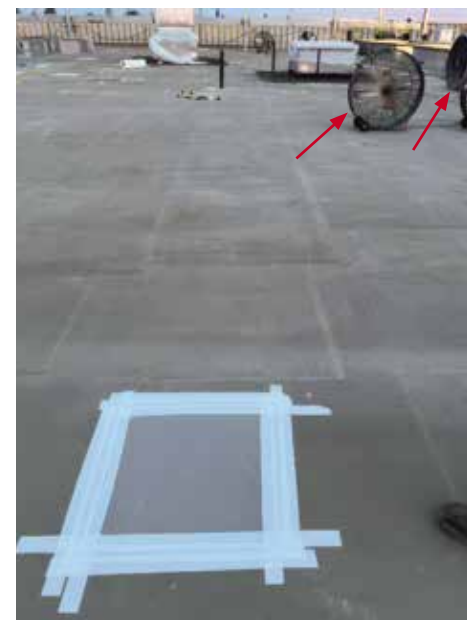
Figure 3. Fans added around concrete for dehumidifying purposes (shown by red arrows).
