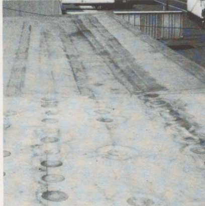
Photo 8 Corner repair with strips and individual fastener repairs with round patches.
