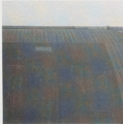
Photo 1 Hanger project installed in 1979. The manufacturer carried out frequent repairs to perimeter and barrel shoulders for the first four years of the installation.
