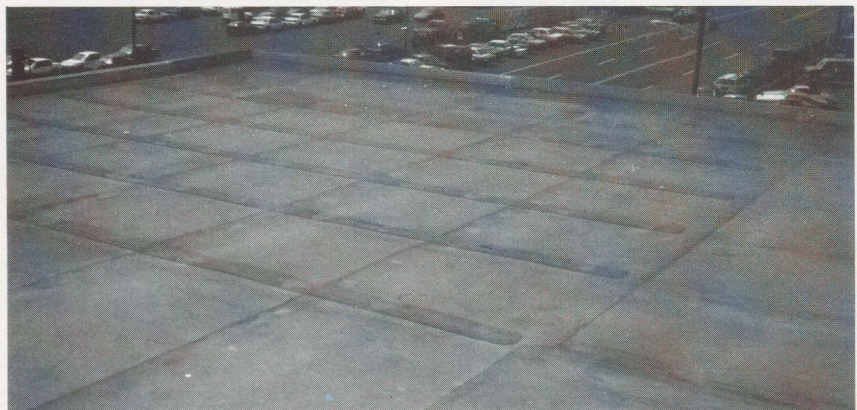
Photo 18 Subsequent corner repair meeting area calculation of ANSI A58.1.
