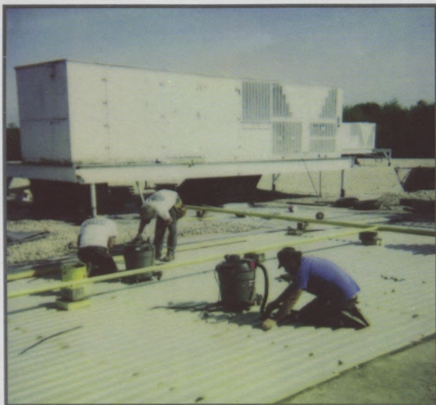
Removal of all foreign materials from deck area.
