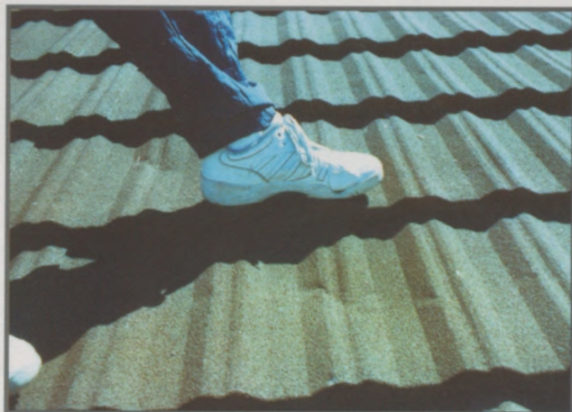
Proper foot position on metal tile panels.
