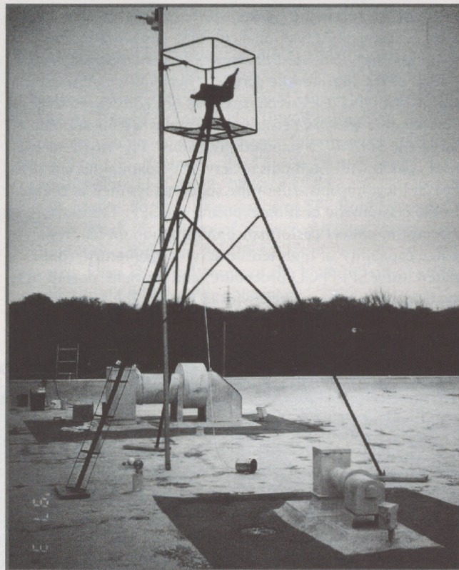
Figure 9: Oversized hail equipment being tested on polyurethane-coated SPF roof system in Dallas, Texas.
