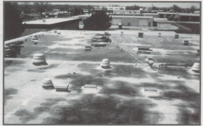
Figure 1: Typical performance-based SPF roof systems in heavy hail areas of Wyoming with 100% customer satisfaction based on 1997 Customer Evaluation Surveys conducted by PBSRG, Arizona State University.
