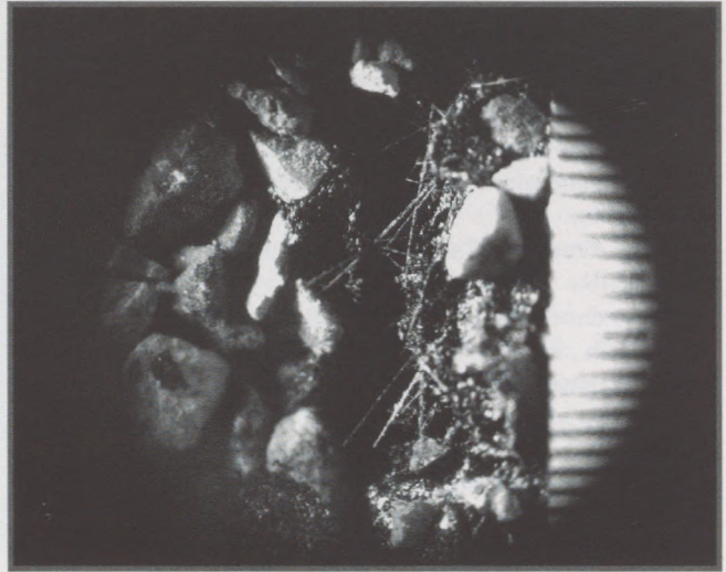
Severe hail: surface fracture damage.
