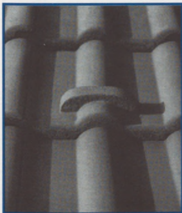
Many European tile manufacturers make field tiles with snow stops as part of the tile.
