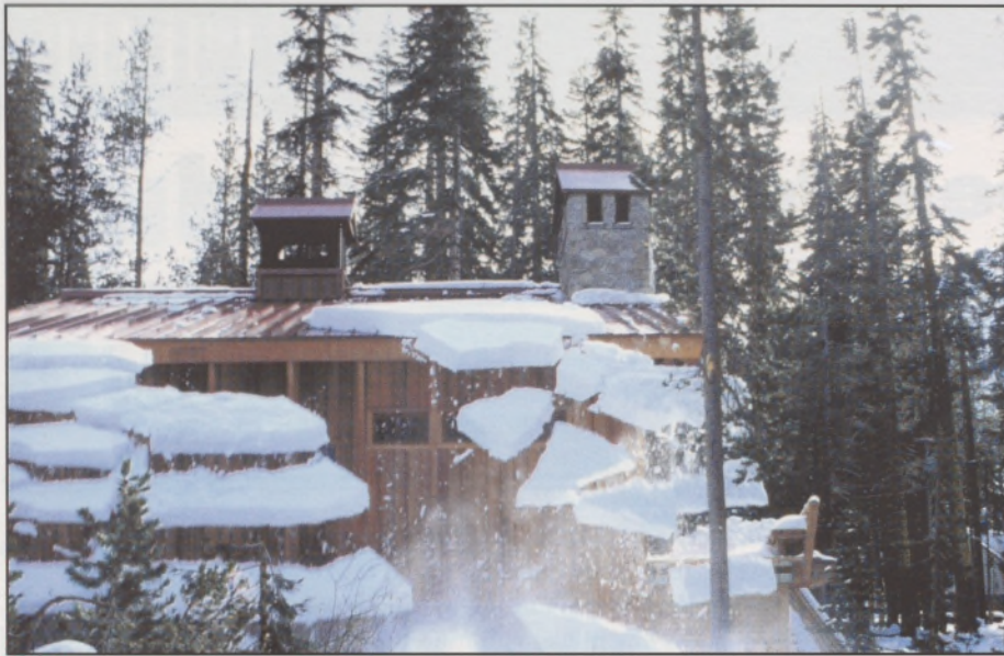
Rick Flood had just come down from the roof of the Hewlett Cabin, in Sugar Bowl, CA (Donner Pass, at 2040' elevation) on Nov. 13, 1998 and gotten out his camera to record a 15" snow-load when the snow cascaded off the roof as he released the shutter. Cold roofs work! © Rick Flood
