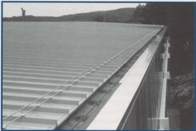
Figure 11: A sure-fire design on IBM's world headquarters incorporates snow retention above an internal gutter which is EPDM lined and heat-traced. The dark color of the rubber and the self-regulating heating cable ensure that the gutter will remain unobstructed and freely draining.
