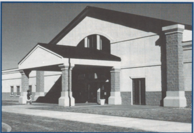
Figure 12: Architectural geometries which place roofs adjacent to higher walls result with the design snow load on such roofs being much greater than ground snow. (due to the "shadow" or drift condition which can accumulate very significant depths of snowbank).
