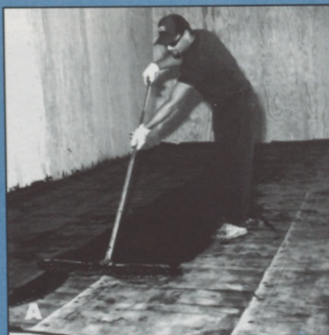
Figure A (left)—Adhesive is applied using a V-notched squeegee.
