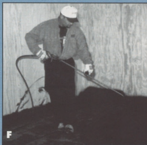
Figure F—Spray application is even faster than a squeegee.
