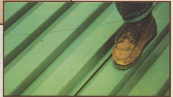
FIGURE 7. CONVENTIONAL STEEL DECKS DO NOT DEVELOP FULL DIAPHRAGM CAPABILITY UNTIL SIDE LAP STITCHING SCREWS ARE IN PLACE.
