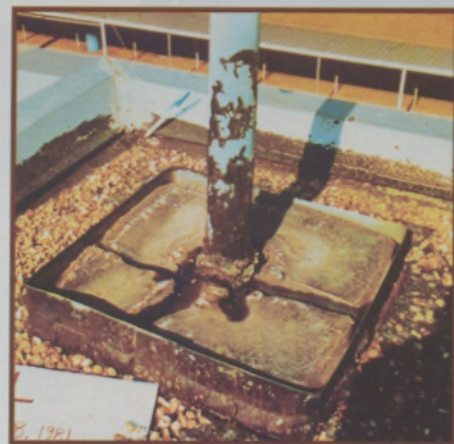
FIGURE 3. RIGID FILLER IN A PITCH POCKET ATTRACTS AND TRANSMITS MOMENT BETTER THAN A RESILIENT PRODUCT. SUSCEPTIBILITY FOR SPLITTING AND SEPARATION THEN BECOMES APPARENT.
