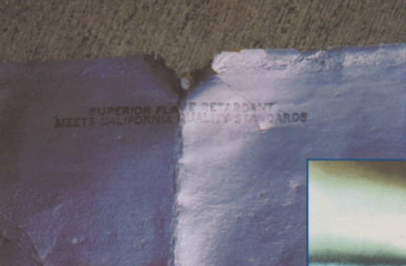
TYPICAL CEILING FOIL PAPER STAPLED BENEATH SUB-PURLINS
