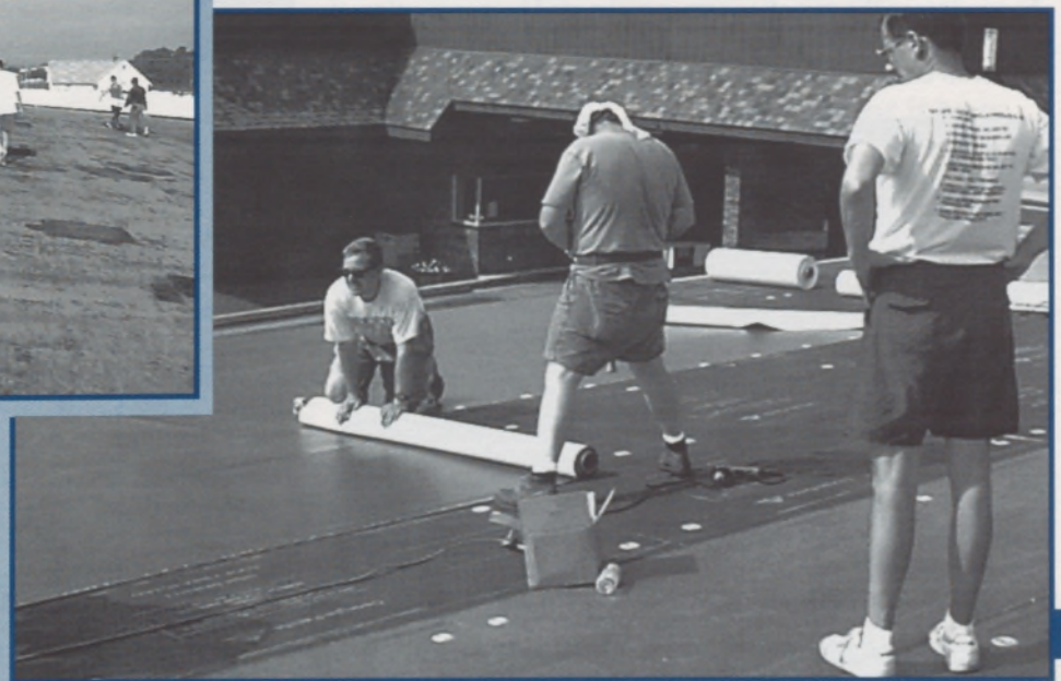
Above: Applying the re-cover insulation. Wood fiberboard was used along the roof, and polyisocyanurate foam along the ridge. Right: Rolling out the black-colored Stevens EP roofing.
