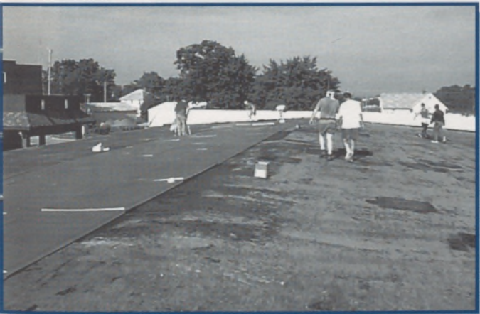
Above: Applying the re-cover insulation. Wood fiberboard was used along the roof, and polyisocyanurate foam along the ridge. Right: Rolling out the black-colored Stevens EP roofing.
