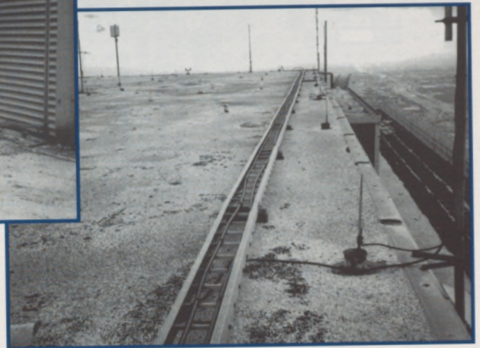
Below: Upper roof after renovation.
