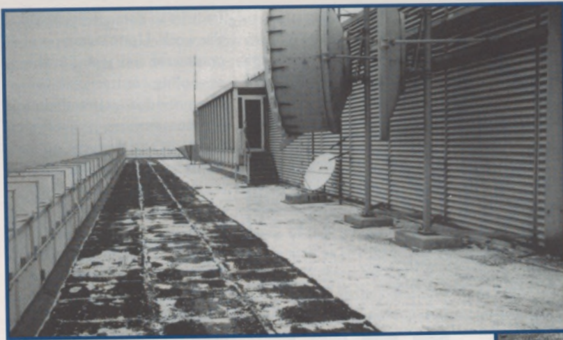
Left: Lower roof prior to re-roof.
