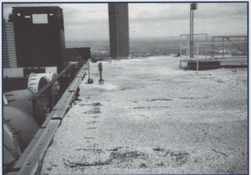
Upper roof after renovation.
