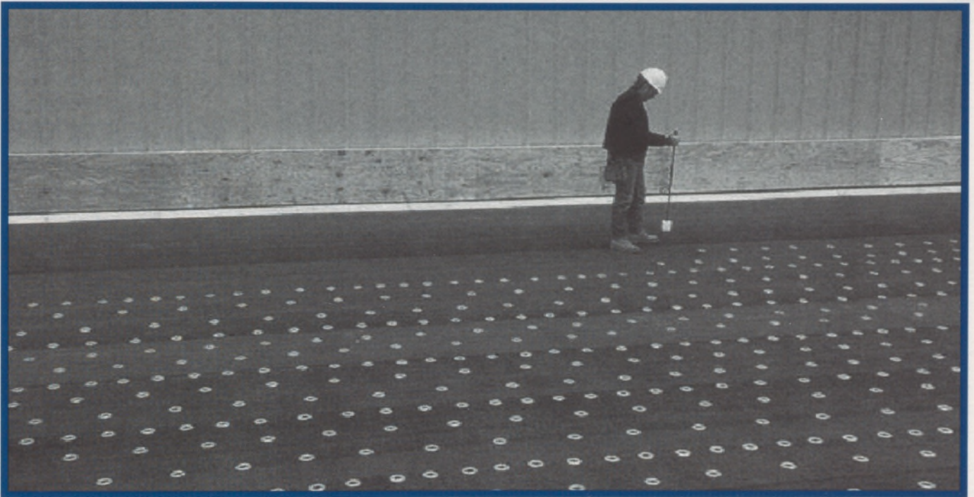
Nailing the base sheet to a lightweight insulating concrete deck.
