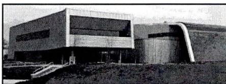
Figure 8 - Solar wall at the main elevation of OptIC, showing the cantilevered business center and 1,000m 2 PV wall array.
