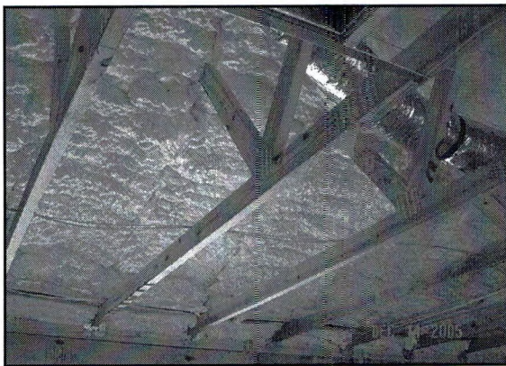
Figures 12A and 12 – Warm- and humid-climate, air-impermeable insulation at the underside of roof-deck application (above). Warm- or mixed- and dry-climate, air-permeable insulation at the underside of tile roof deck application (right).
