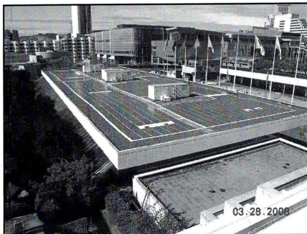
Figure 1 – Large array of photovoltaic panels installed on a roof in San Francisco.
