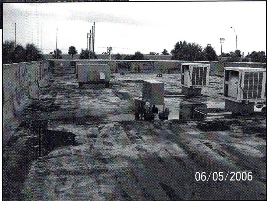
Figures 3 and 4 – Examples of natural weathering observed on a flat-roof system.
