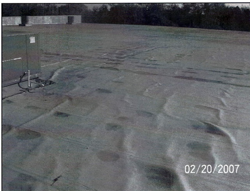
Figure 6 – Example of wind uplift damage to a portion of a smooth-surfaced modified-bitumen roof membrane.
