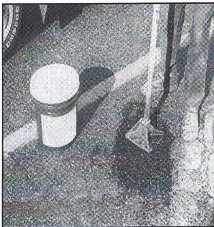
Figure 5 - Asphalt patching compound produced from postconsumer vinyl membranes and other recycled plastics.
