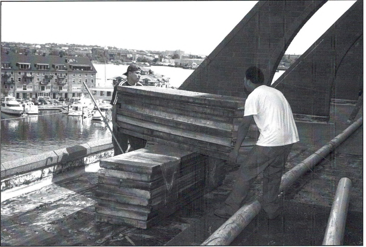
Figure 9 – Extruded polystyrene insulation being saved for reuse.
