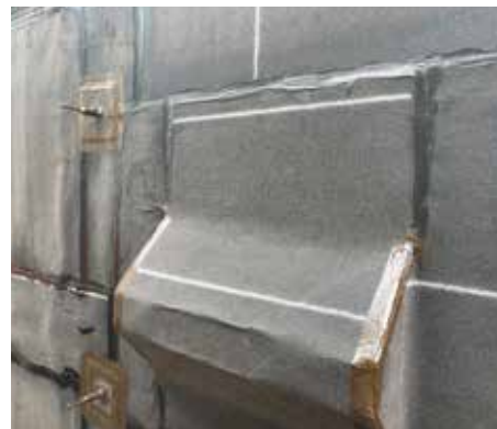
Figure 16. Styrene butadiene styrene modified bitumen waterproofing installed.
