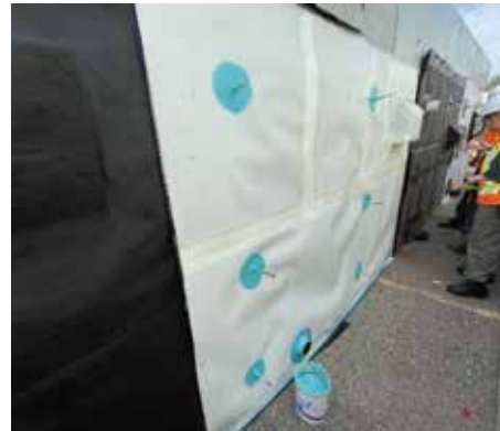
Figure 14. High-density polyethylene sheet waterproofing installed.
