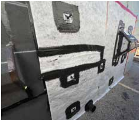
Figure 13. Elastomeric sheet waterproofing installed.
