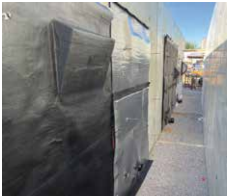
Figure 15. Elastomeric spray applied waterproofing installed.
