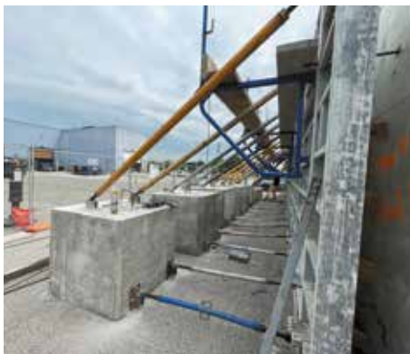
Figure 17. Formwork in place for pouring of concrete from bucket.
