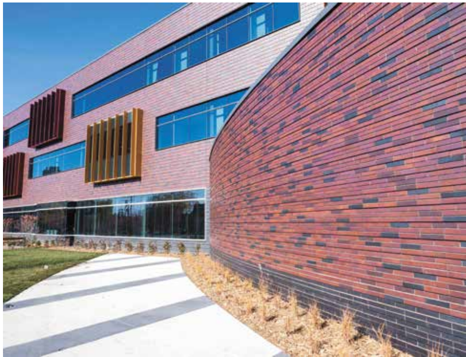
Figure 7. Precast insulated sandwich wall panels can utilize thin brick in a variety of colors and coursing patterns to achieve a wide range of looks.
