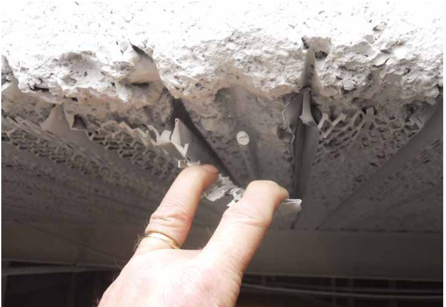
Figure 7. Longer spans (that is, greater spacing of supports) could result in sagging between supports, so bar reinforcing was added to strengthen the section. Smooth bar shown here evidently predates the diamond pattern of modern “deformed” bars, which were first used in the 1920s.
