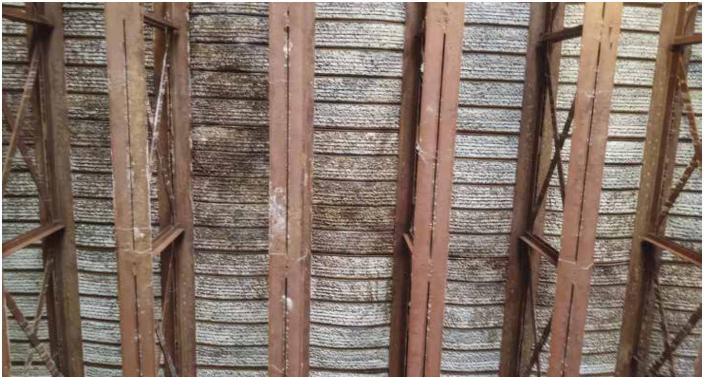
Figure 3. When cinder concrete was in vogue, it was likely to have been used as the floor construction as well. Here the closer spacing of floor framing distinguishes it from that which would be found at the roof level.
