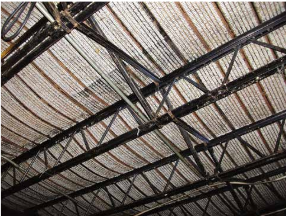
Figure 1. Cinder concrete is a type of cast-in-place mix, placed atop ribbed and expanded metal form (also known as wire lath). This support system was used for concrete floors before the advent of modern ribbed/fluted steel form deck.
