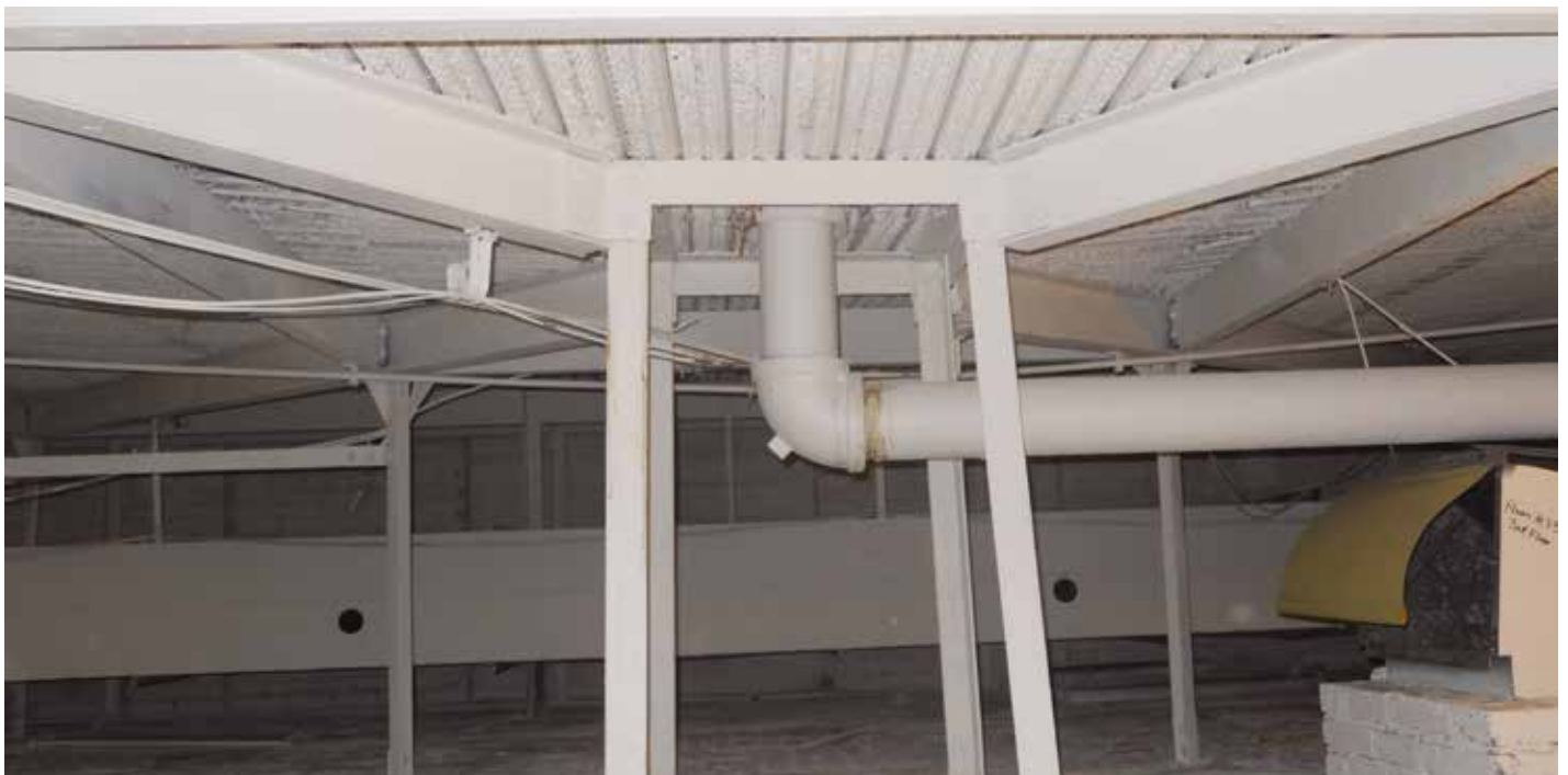
Figure 8. Supplementary steel framing is needed in locations similar to other deck types. Here steel bracing has been provided for a roof drain opening.
