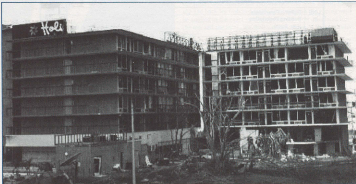
Figure 6: Florida high-rise destruction during Hurricane Andrew (photo ©1992 Roger Edwards).
