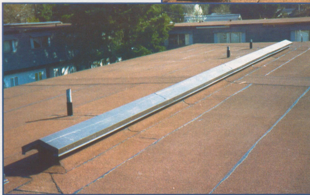
(above) Ridge vent and finished roof.
