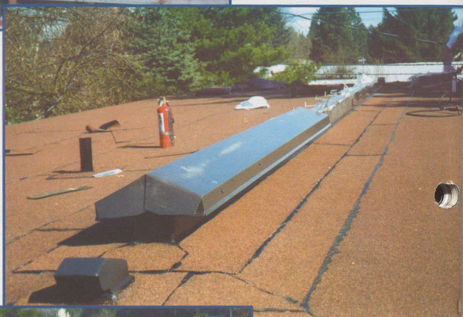
(above) Ridge vent and finished roof.
