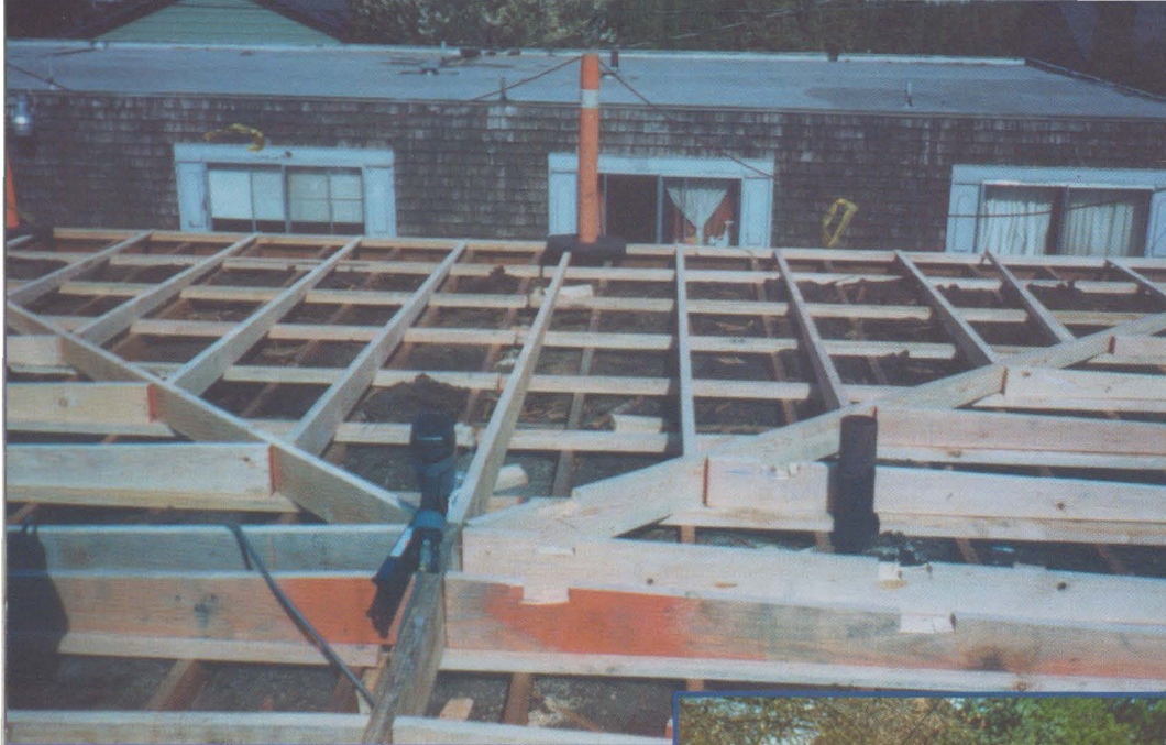
New rafters leading to center ridge vent.
