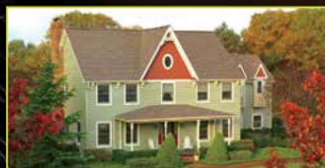
Residential "Cool" Roofing
