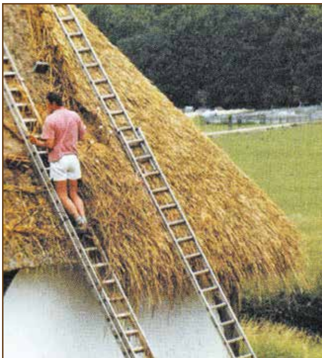
Photo 7 – The hall from Boarhunt being thatched with long straw.
