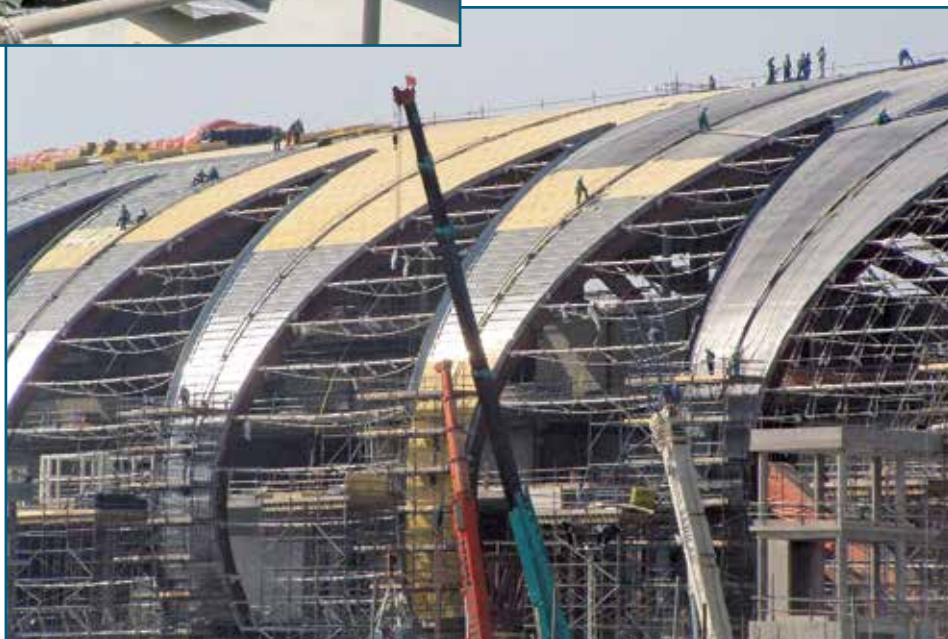
Figure 6 – Crane lifting secondary components to the roof level. Special on-roof support platforms were required.
