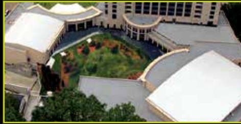
White Asphaltic Roofing
