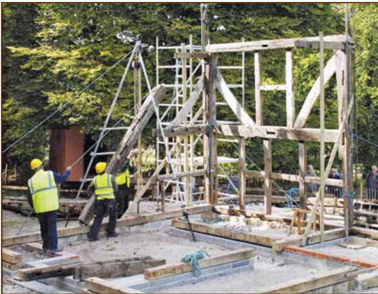
Photos 10 and 11 – The reassembly of the 17th-Century cottage oak frame commenced in September 2012 and has attracted many visitors to the museum.
