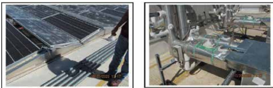
Figure 11. The solar panels were destroyed by hail, and the fractures in the panels were in the 2.5 in. (64 mm) to 3 in. (76 mm) range.
