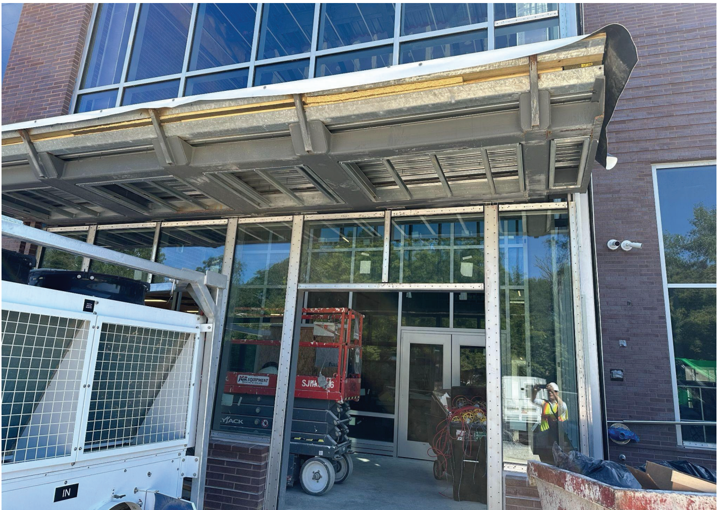
Figure 3. Canopy transition condition that is frequently a source of air leaks during a whole building airtightness test.
