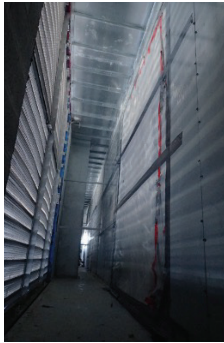
Figure 6. Two different plenum shafts where the interior wall must be sealed as part of the air control layer.
