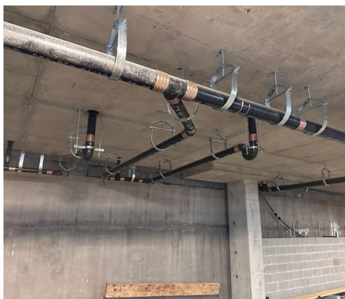
Figure 4. Penetrations through the wall of a parking structure that must be sealed airtight to complete the building's continuous air barrier.
