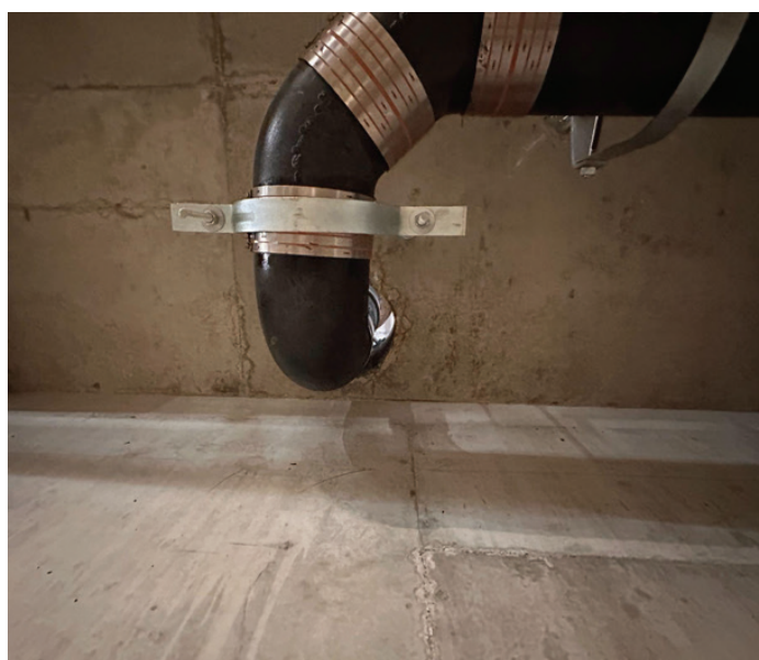
Figure 4. Penetrations through the wall of a parking structure that must be sealed airtight to complete the building's continuous air barrier.
