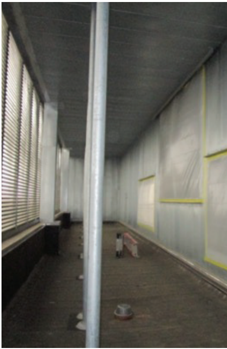
Figure 6. Two different plenum shafts where the interior wall must be sealed as part of the air control layer.
