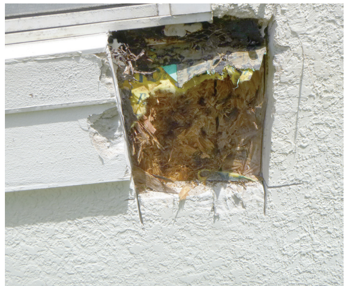
Figure 4. Example of damage resulting, at least in part, from improper separation between window and stucco, violating ASTM C1063 7.11.7 and ASTM C926 7.3.4, A2.1.2, A2.1.3.
