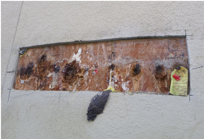
Figure 1. Example of damage resulting, at least in part, from fasteners installed between framing members, violating ASTM C1063 7.9.1, 7.10.2.2.
