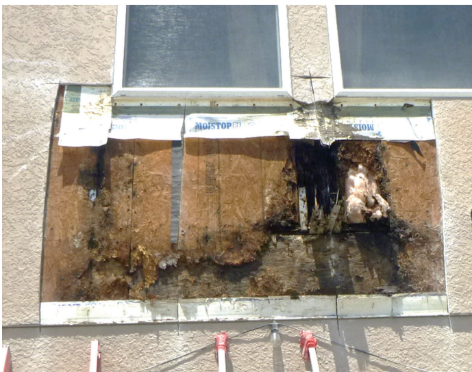
Figure 5. Example of damage resulting, at least in part, from improper separation between window and stucco, violating ASTM C1063 7.11.7 and ASTM C926 7.3.4, A2.1.2, A2.1.3.
