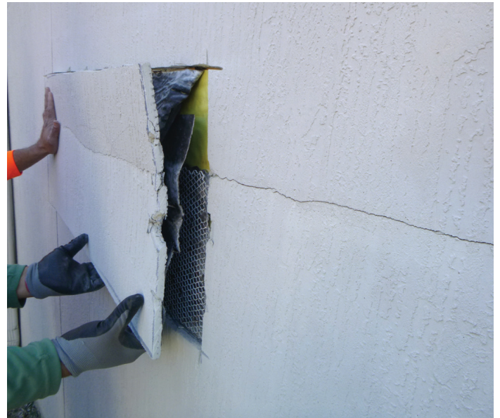
Figure 2. Example of damage resulting, at least in part, from lath not installed backing on backing and metal on metal, violating ASTM C1063 7.9.3.
