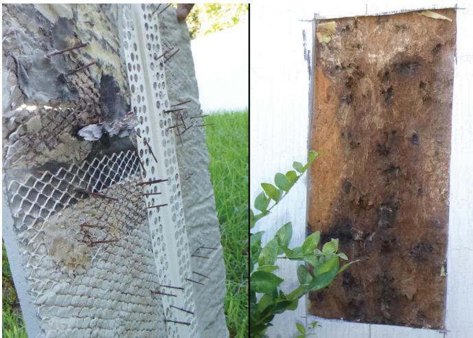
Figure 3. Example of damage resulting, at least in part, from the fastening down of the control joint accessory, violating ASTM C1063 7.10.1.5.
