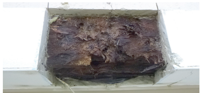
Figure 6. Example of damage resulting, at least in part, from a missing weep accessory at the horizontal-to-vertical intersection, violating ASTM C926 A2.2.2.
