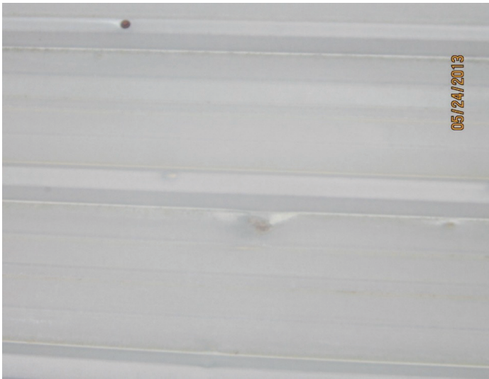
Figure 10. Photograph of the dents in the case study roof caused by the Mayfest Storm.
