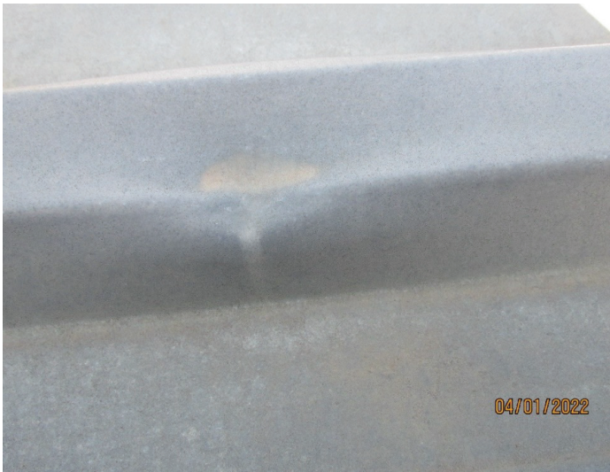
Figure 15. Photograph of large dent in the rib of the panel.
