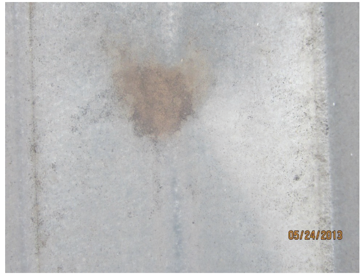
Figure 11. Photograph of typical hail-caused indentations with stains in the dents.
