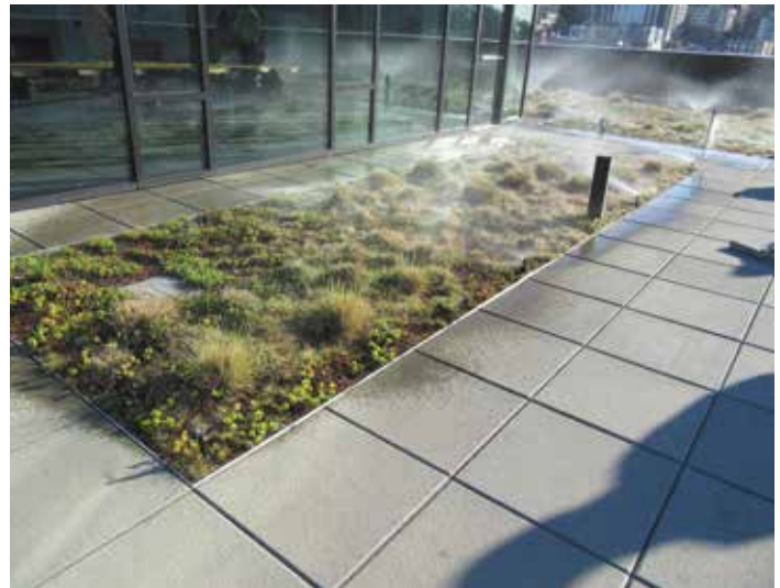
Figure 8. The three vegetative roof areas at the southern end of the eighth-floor roof were saturated with water from the irrigation system, which replicated the leak for the first time (3/16/2020).
