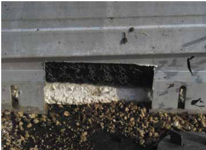
Figure 11. Southeast vegetative roof area was discovered to have expanded polystyrene (EPS) insulation resting directly on the roofing membrane, with the drainage composite installed over the EPS insulation (3/18/2020).
