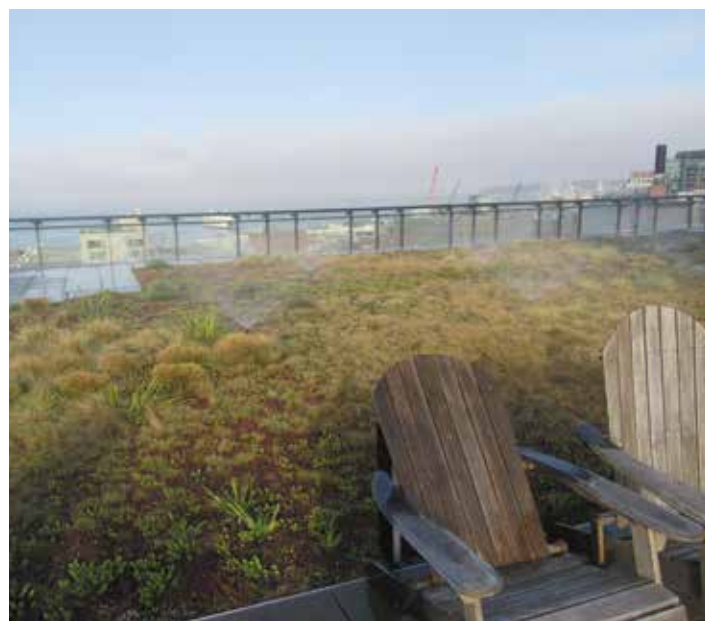
Figure 10. Saturating the southwest vegetative roof separately did not replicate the leak (3/18/2020).
