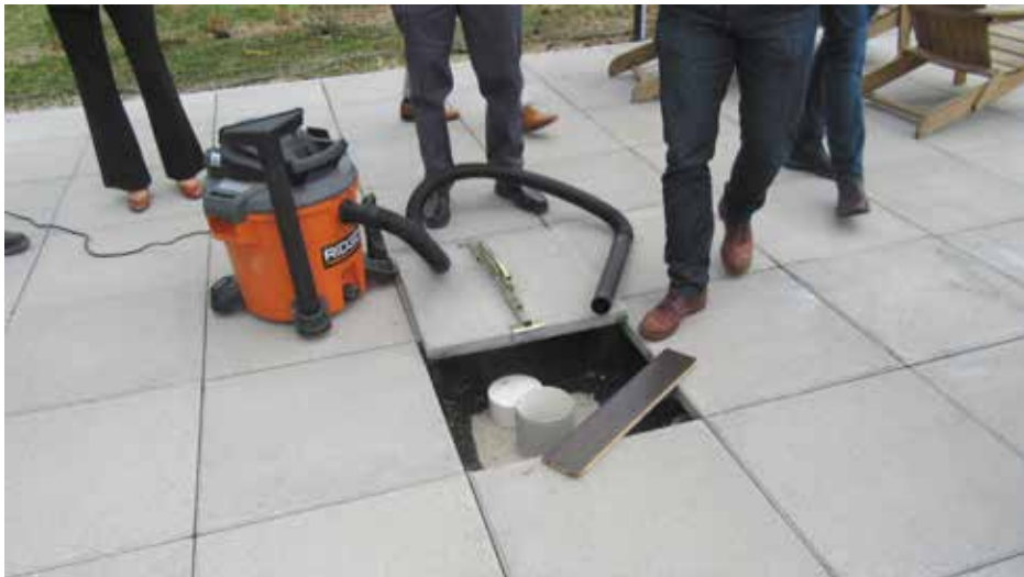
Figure 5. Inspection port installed under pavers on pedestals at south patio area of eighth-floor green roof (2/17/2019).
