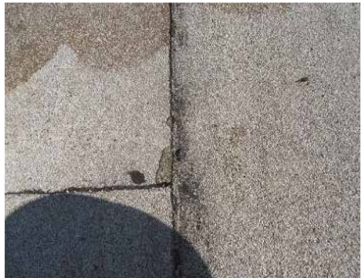
Figure 22. Additional water seepage from the roofing seam subsequent to the time recorded by Figure 20 (7/29/2020).
