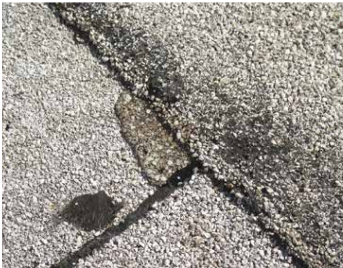
Figure 21. Close-up view of water seeping out of the roofing seam (7/29/2020).
