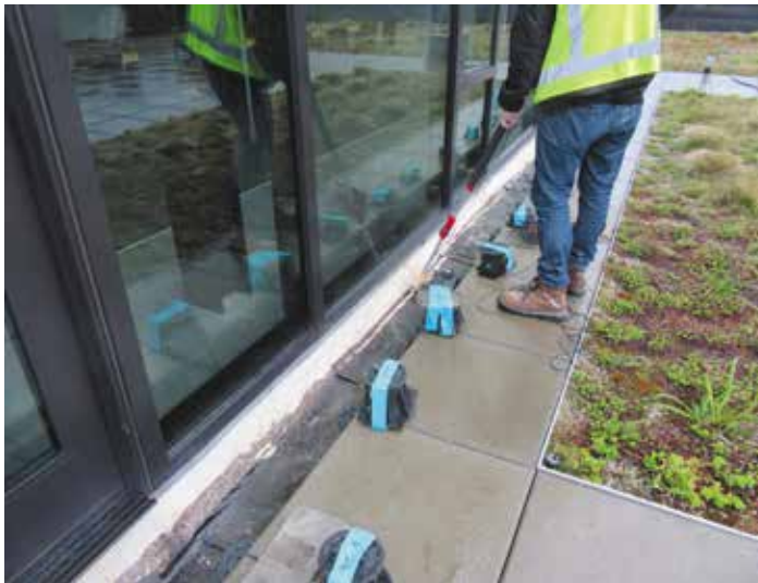
Figure 7. Electronic leak detection was used to confirm no breaches in base flashing membrane along the base the penthouse structure (3/02/2020).
