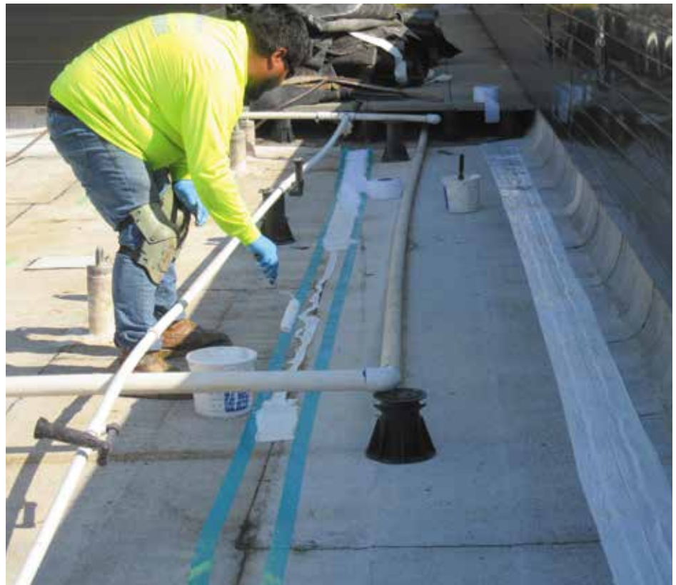
Figure 23. Polymethyl methacrylate flashing membrane being applied to all roofing seams in the southeast vegetative roof area (8/05/2020).
