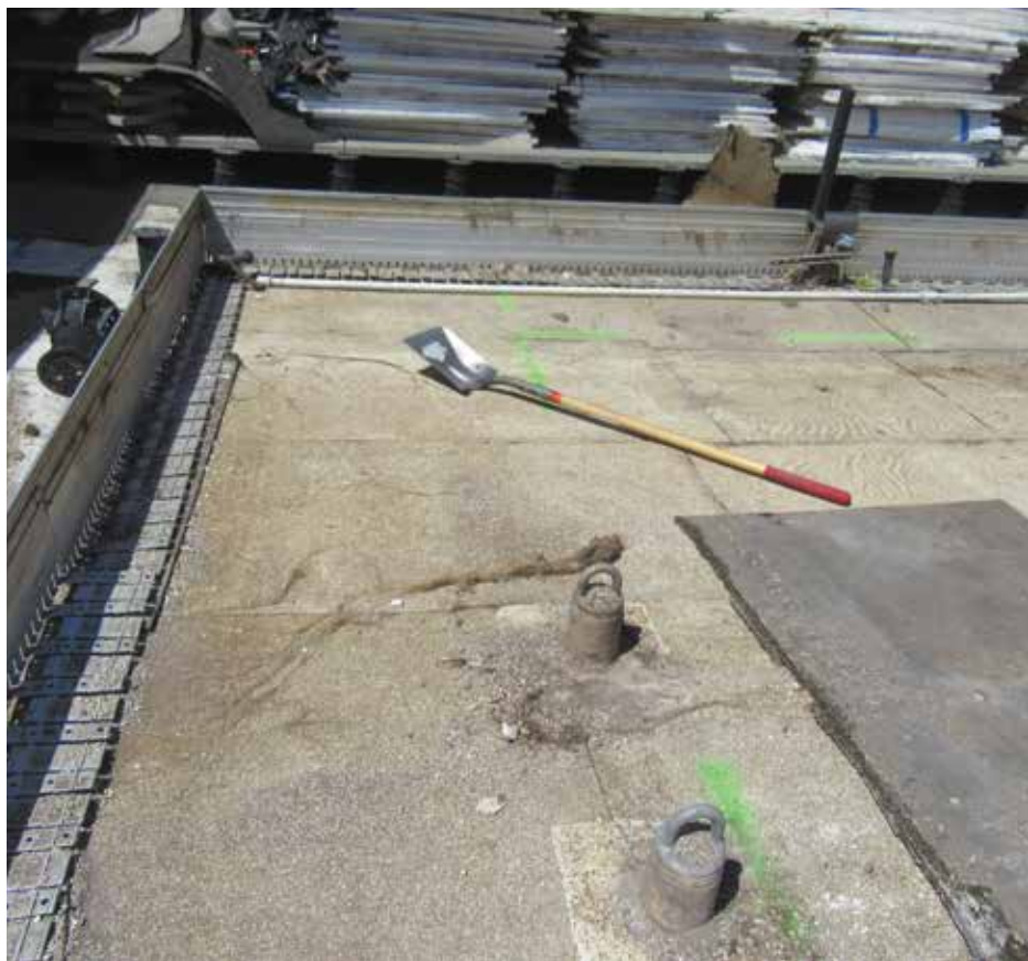
Figure 17. Vegetative assembly removed from the southeast corner of the main roof. Minor root growth was discovered to have penetrated the root barrier but without evident damage to the roofing membrane (7/14/2020).
