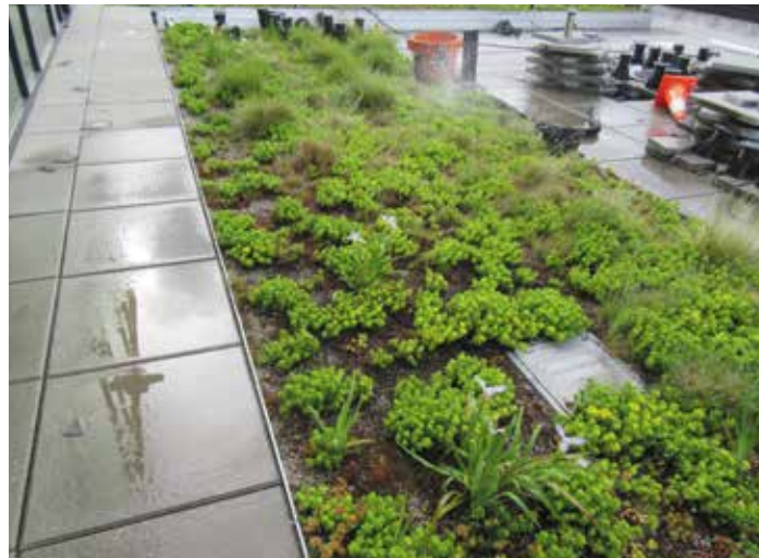
Figure 16. South-central vegetative area was also water tested separately, but it did not replicate the leak despite having expanded polystyrene insulation resting directly on the roofing membrane (5/22/2020).
