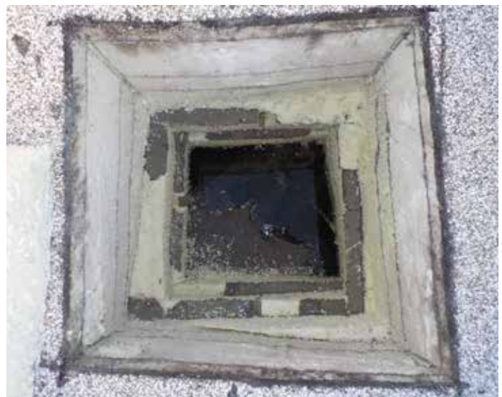
Figure 4. Exploratory opening revealing water at the level of the roof air/vapor barrier, but no breaches (2/02/2017).
