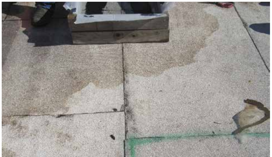
Figure 20. General view of roofing membrane upslope of flood test location with water visibly seeping out of the T-lap seam (yellow circle) (7/29/2020).
