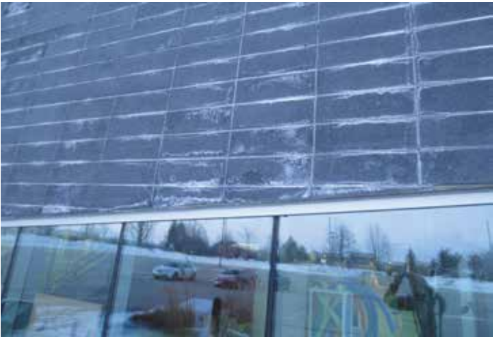
Figure 16. Around the windows, there was greater mortar damage and efflorescence as a result of the lack of deficient air barrier details.
