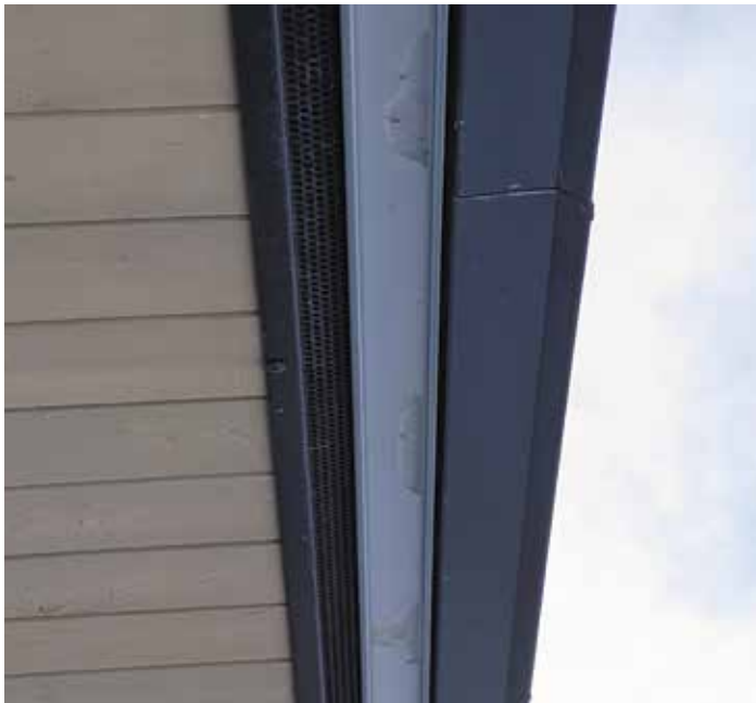
Figure 13. Photograph of water within the light fixtures at the edge of the soffit.
