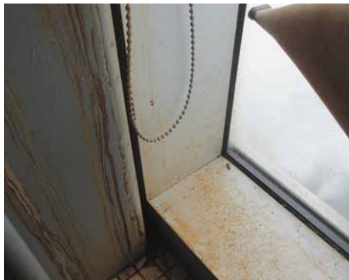
Figure 8. Staining inside the pool area running down steel columns from the parapet.
