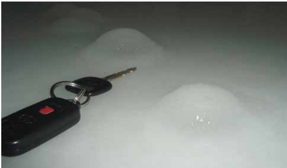
Figure 6. Mounding on ice formed when air leaked from the common areas and the pool leaked into the ceiling above the ice rink, condensed, and dripped onto the ice.
