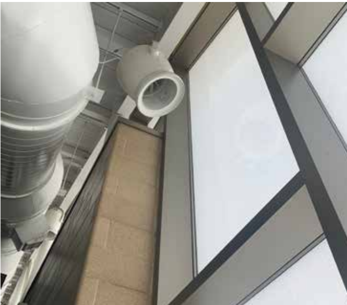
Figure 14. Fans were added during the building repairs to blow air directly over the windows to reduce condensation on the interior surfaces of the windows.
