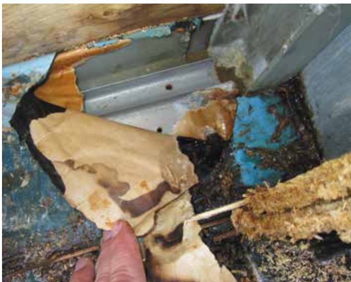
Figure 7. Water accumulation and damage in the parapet, and the backer observed on the Blueskin air barrier.
