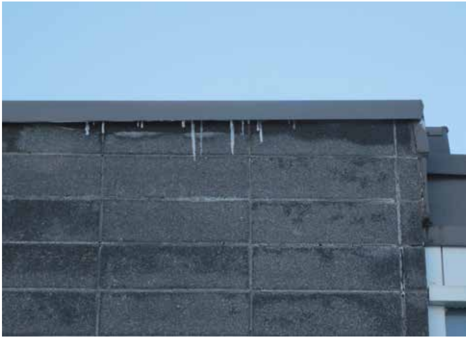
Figure 17. At the top of the wall, icicles, wetting, efflorescence, and mortar damage were all present as a result of air leakage.
