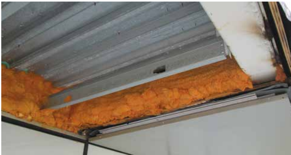
Figure 10. Closed-cell spray polyurethane foam (ccSPF) was installed above the windows at the transition between the metal roof deck and the enclosure over the green fluid-applied air and water barrier. ccSPF was also installed around the entire length of the HSS supporting the soffit and connected to the interior structure to minimize thermal bridging.
