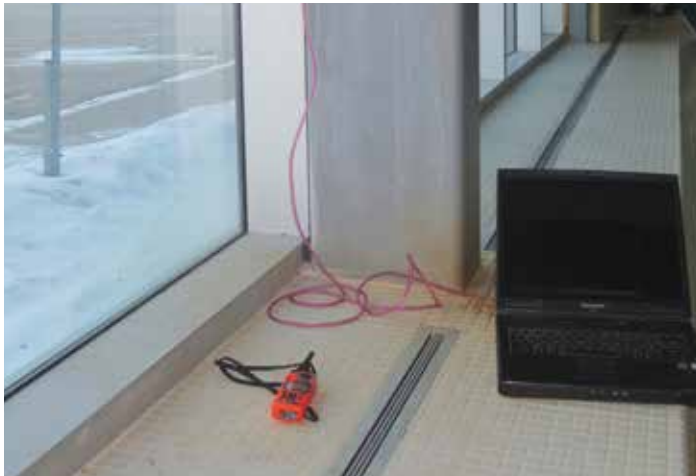
Figure 15. Linear grilles adjacent to the windows are designed to apply airflow to the window area, reducing condensation.
