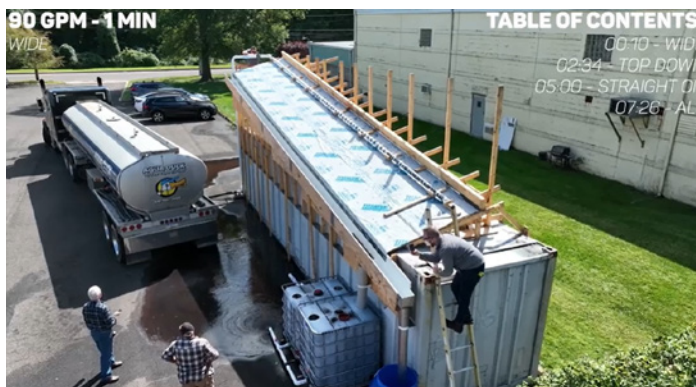
FIGURE 14. Overview of performance mock-up. Note the complex geometry of the roof slope and steep-slope gutter.
