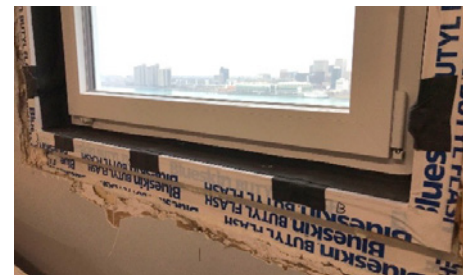
FIGURE 12. Supplemental interior air barrier application at window perimeter.
