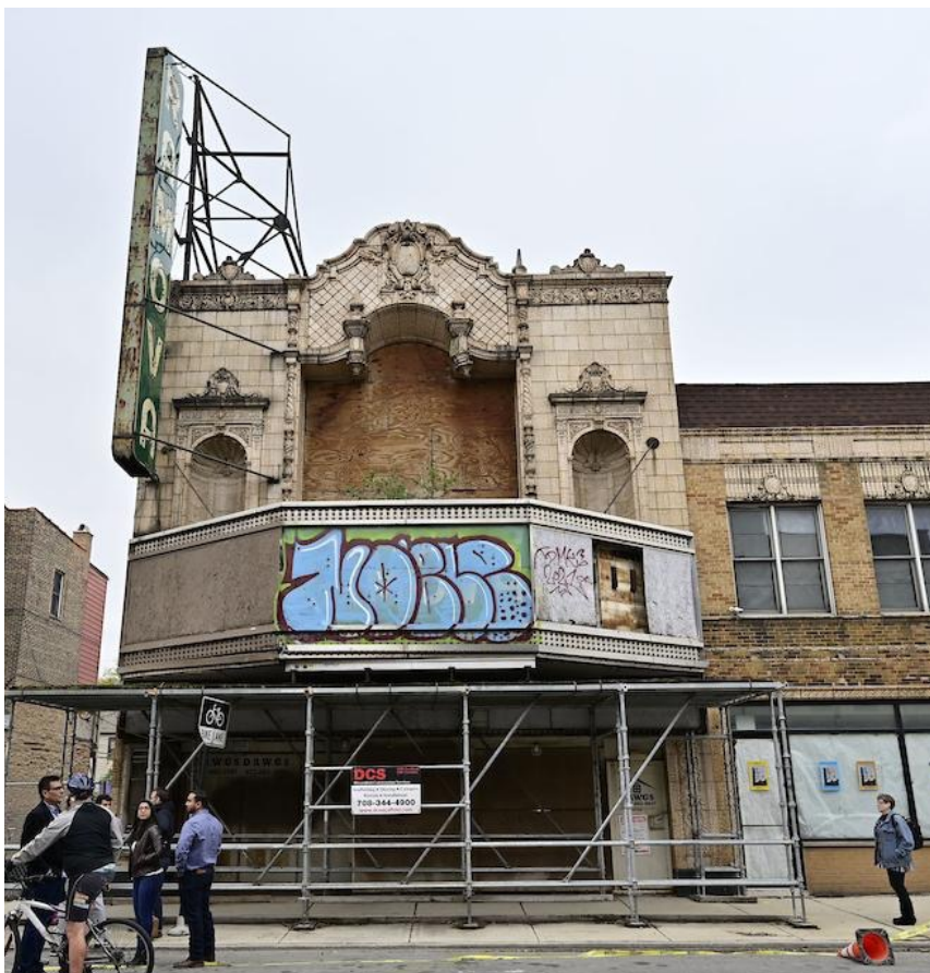
FIGURE 2. View of existing conditions of the east facade elements (terra-cotta, marquee and blade signs, and monumental window) of the Ramova Theatre in spring 2021.
