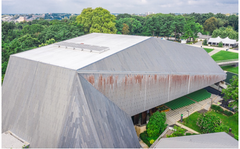
FIGURE 1. Overview of the east elevation of the Mann Center for the Performing Arts from the lawn via a drone survey performed in August 2019.
