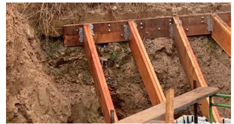
FIGURE 14. The excavation had to be reinforced due to constant water movement below the concrete retaining wall .
