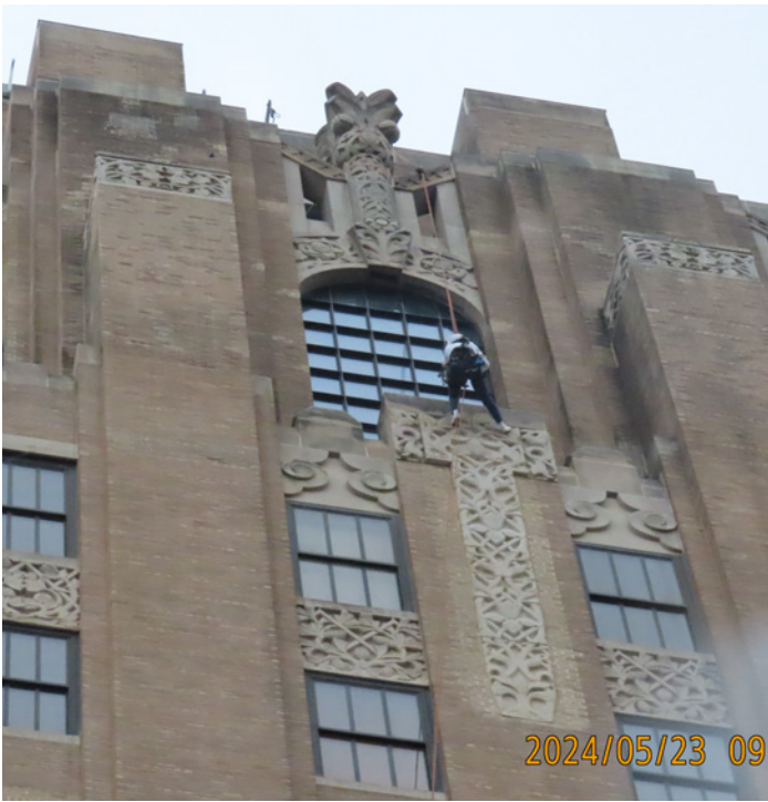
FIGURE 6. Inspector performing facade inspection via industrial rope access. Photograph by Mike Lopez, May 23, 2024. Rimkus.
