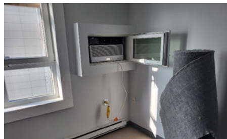
FIGURE 11. Completed window enclosure for the through-the-wall air-conditioning system.
