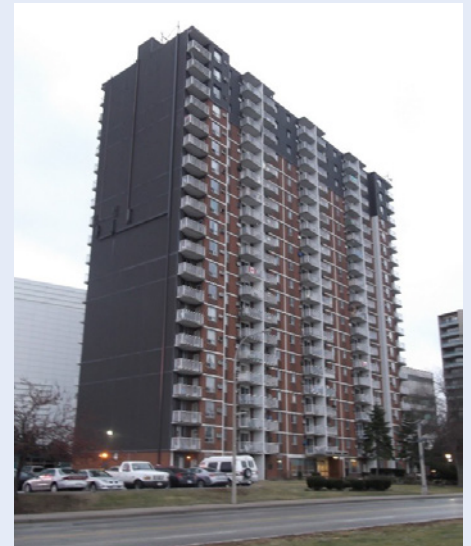
FIGURE 1. 255 Riverside Drive (Raymond Desmarais Manor) before the deep energy retrofit.
