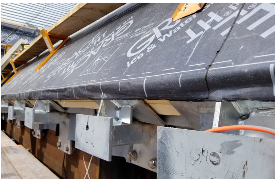
FIGURE 2. Roof edge support in progress.
