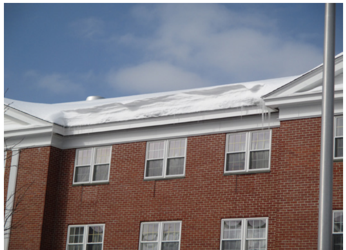
FIGURE 6. Sufficient ventilation, resulting in negligible ice dams or icicles.
