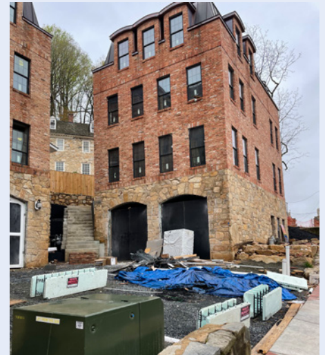
FIGURE 1. Overall view of the subject property during construction.
