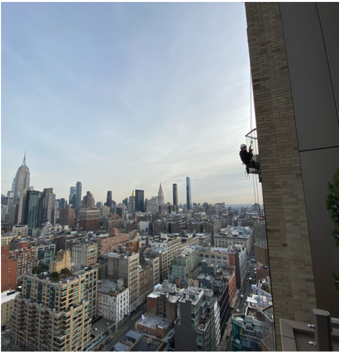
FIGURE 7. Inspector performing facade inspection via industrial rope access. Photograph by Mike Lopez, January 25, 2022. Rimkus.
