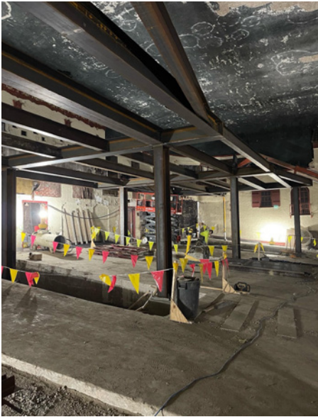
FIGURE 7. View during construction, showing new support steel structure for balcony, including footing repairs and interface with interior plaster.
