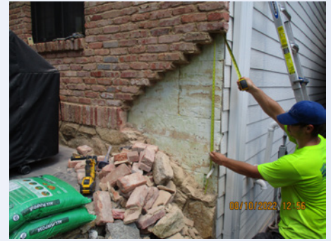
FIGURE 9. Destructive testing was performed to document concealed conditions.
