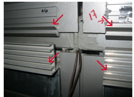
FIGURE 5. Testing of added heat sinks at a four-way glazing system intersection.
