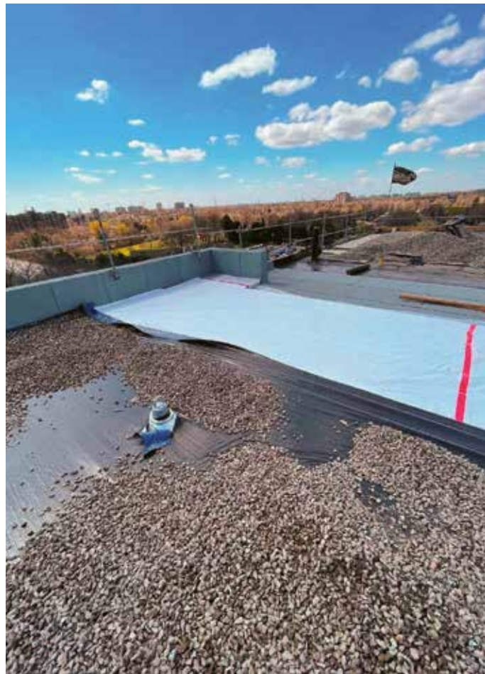
Figure 7. New protected membrane roof system under construction.
