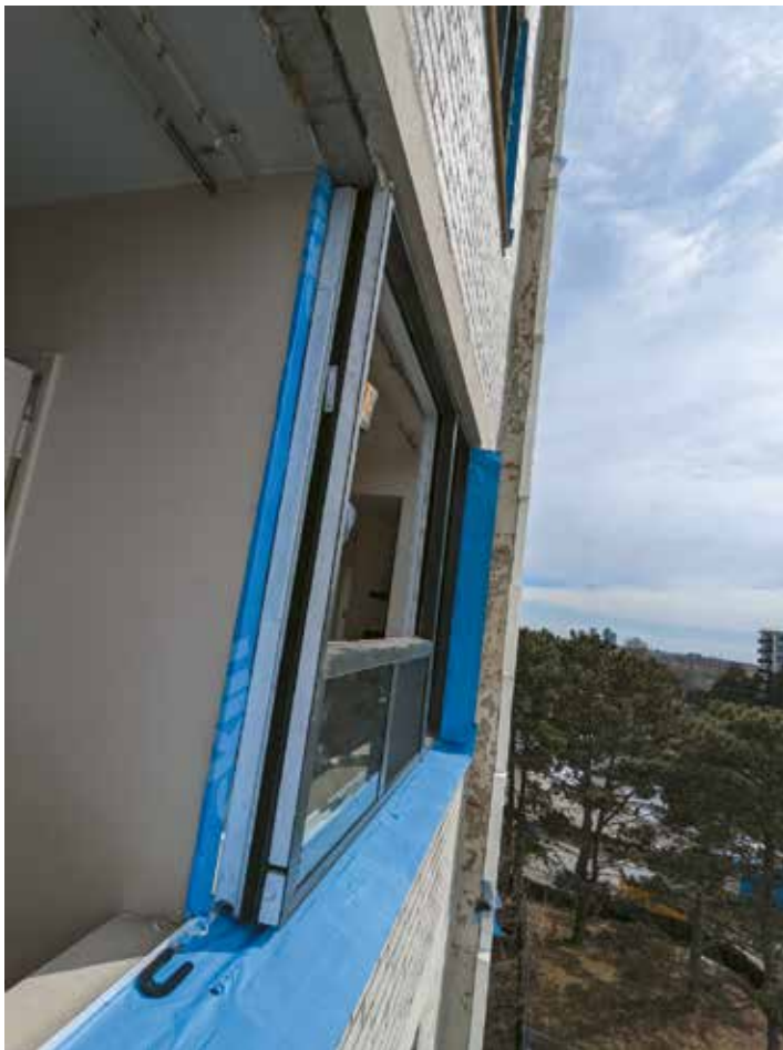
Figure 6. New residential window systems with subsill flashings.
