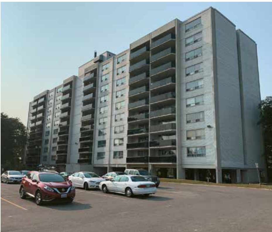
Figure 1. East elevation, preconstruction.
