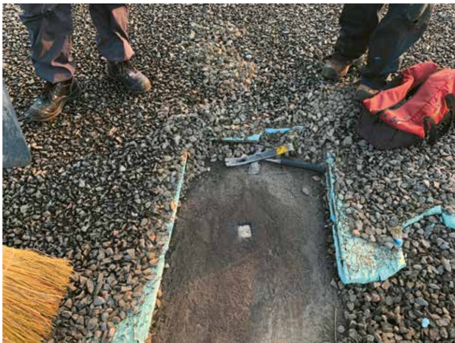
Figure 4. Test cut within existing roofing system.
