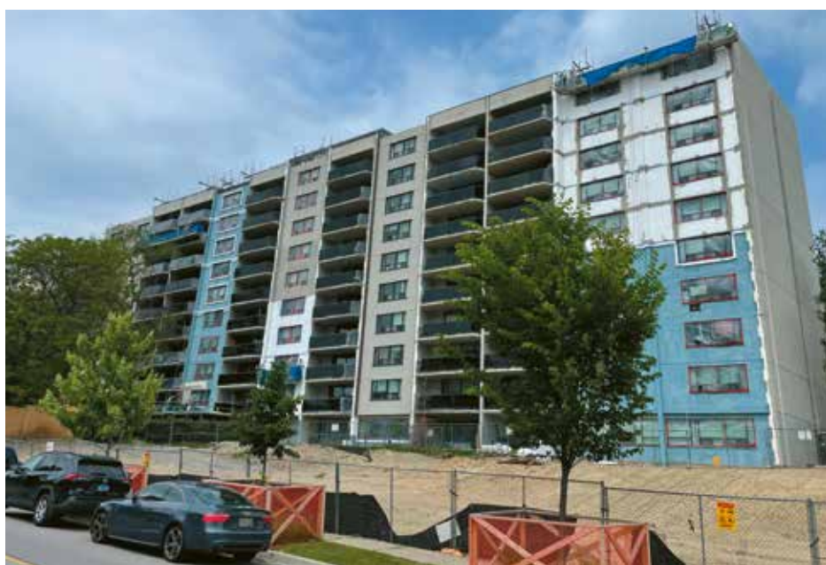
Figure 5. Exterior insulation and finish system installation on the west elevation.
