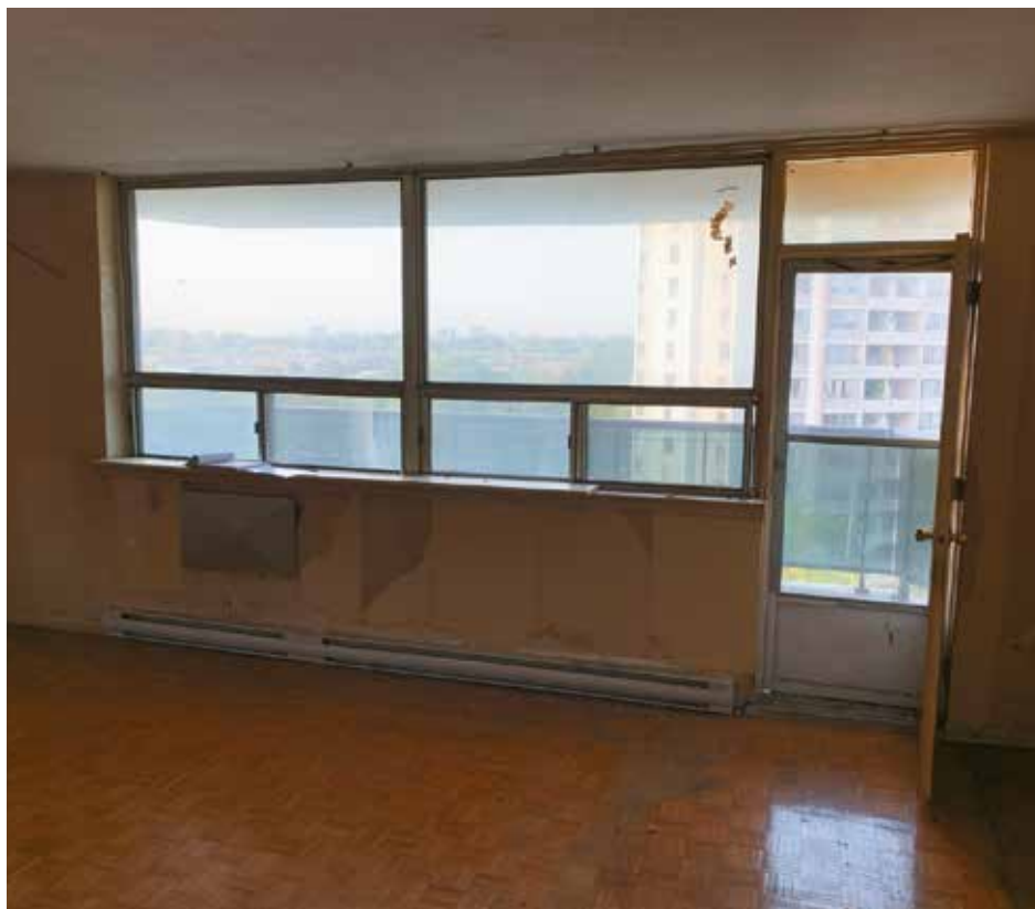
Figure 3. Existing in-suite windows and balcony swing doors.
