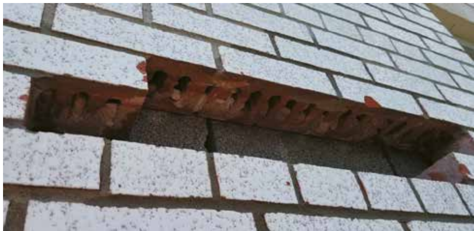
Figure 2. Exploratory opening in brick masonry.
