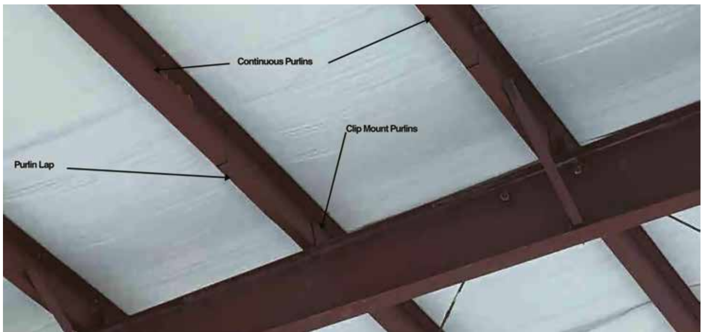
Figure 2. Continuous clip-mounted purlin lap over frame.
