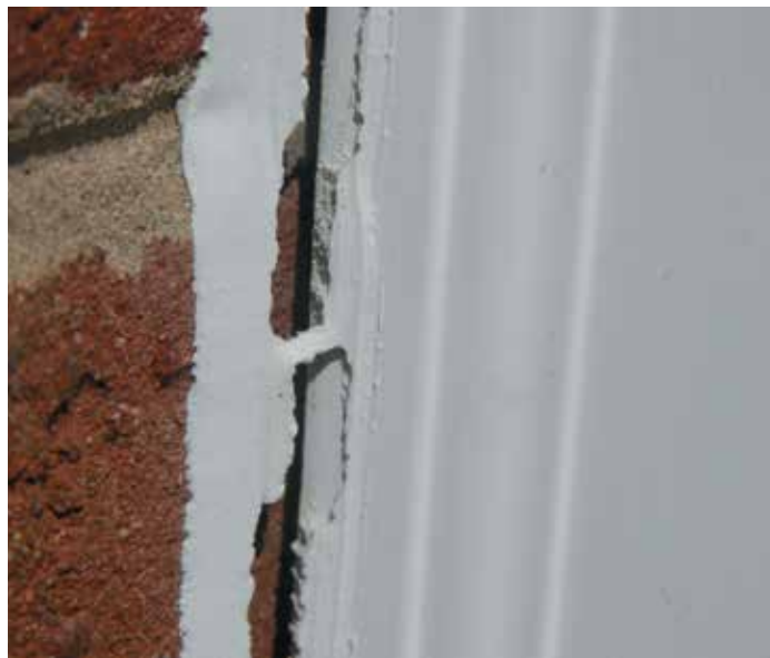
Photo 3. Sealant separation at a window secured to wood framing due to shrinkage of the wood framing and expansion of the brick veneer. Photo from Rimkus Archives.
