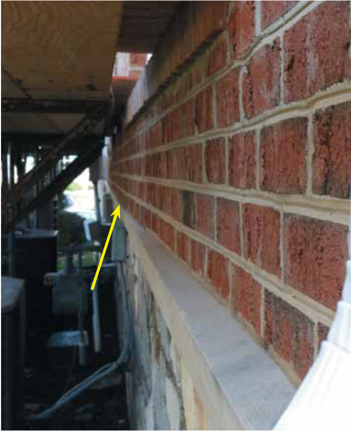
Photo 13. Bowed brick veneer. Photo from Rimkus Archives.
