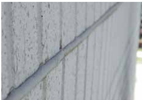
Photo 4. Compressed sealant at a horizontal movement joint. Photo from Rimkus Archives.
