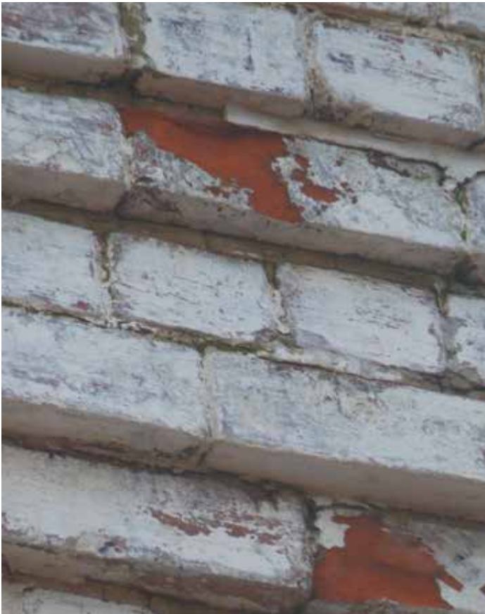
Photo 11. Spalled brick. Photo from Rimkus Archives.
