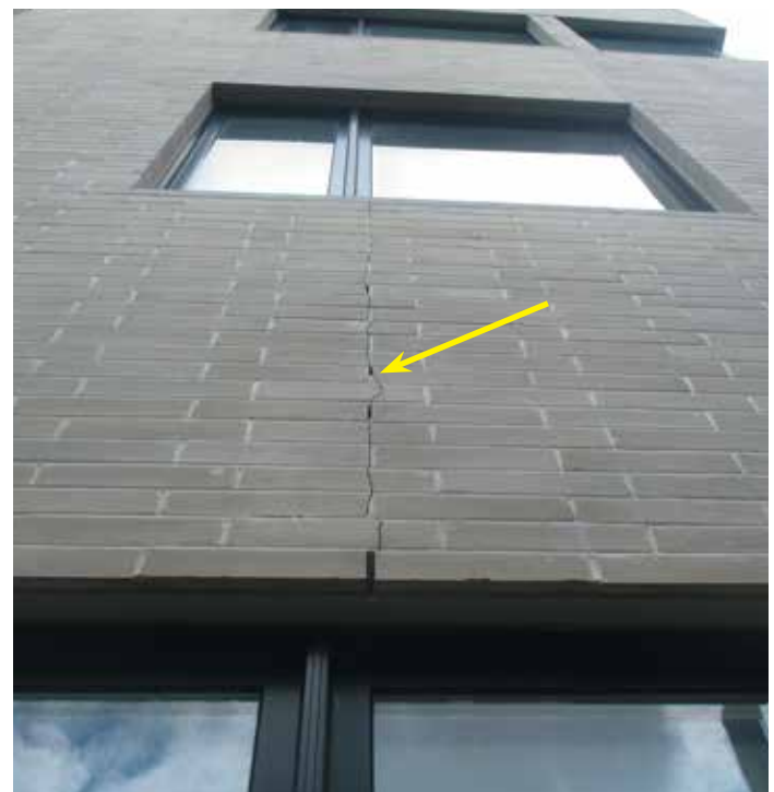
Photo 8. A vertical crack. Photo from Rimkus Archives.
