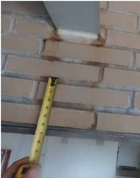
Photo 16. Efflorescence on the brick-and-mortar joint surfaces. Photo from Rimkus Archives.
