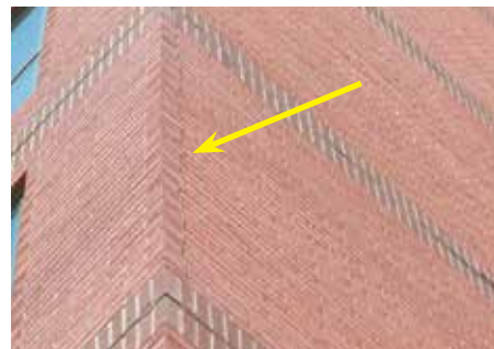
Photo 5. A corner crack in the anchored brick veneer. Photo from Rimkus Archives.
