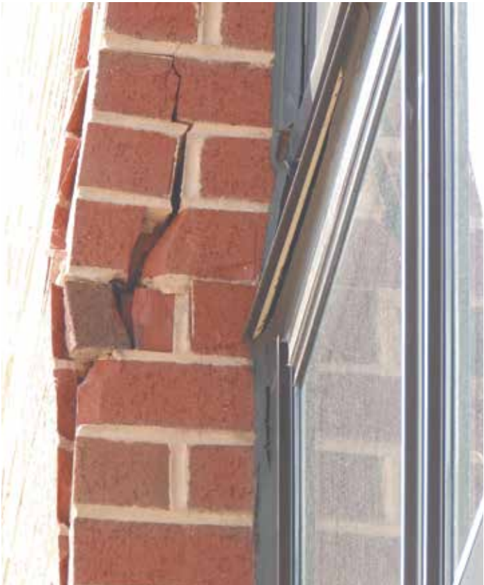
Photo 12. Spalled and fractured brick due to compression. Photo from Rimkus Archives.
