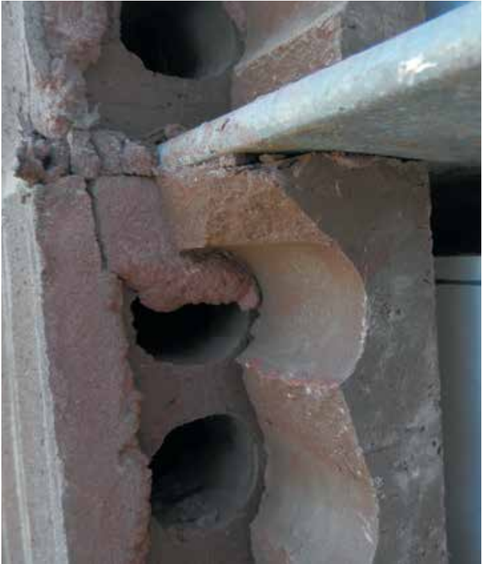
Photo 10. A view of the steel shelf angle below a horizontal crack. Photo from Rimkus Archives.
