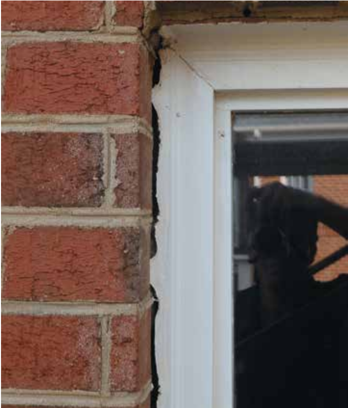
Photo 14. Joint separation at the window in a bowed brick veneer wall. Photo from Rimkus Archives.
