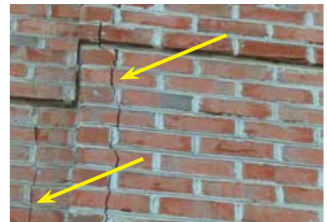
Photo 6. A corner crack in the anchored brick veneer. Photo from Rimkus Archives.
