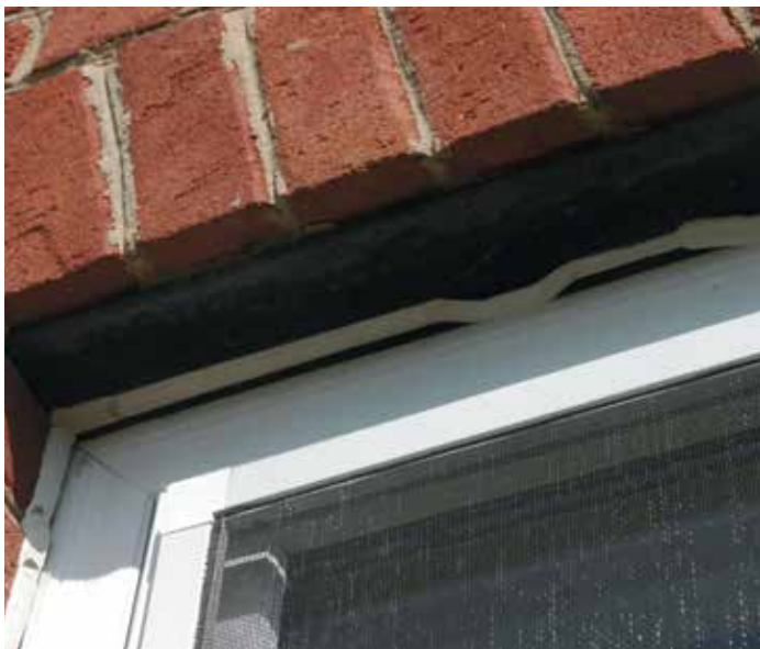
Photo 2. Sealant separation at a window secured to wood framing due to shrinkage of the wood framing and expansion of the brick veneer. Photo from Rimkus Archives.
