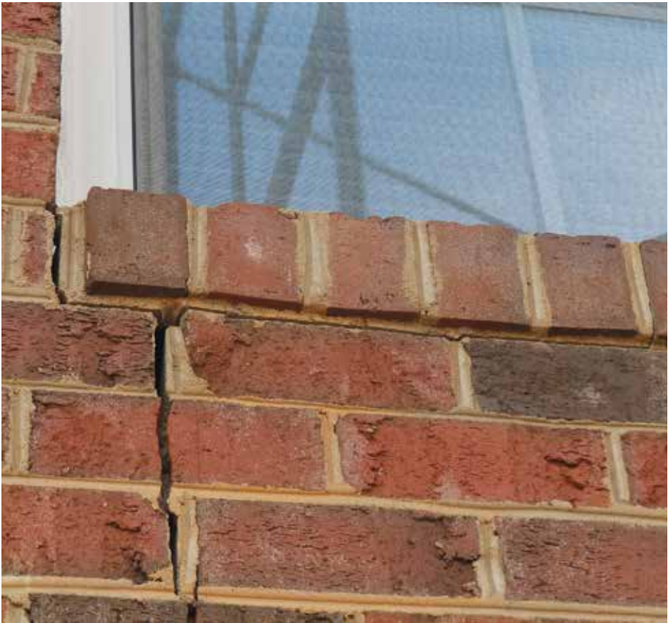
Photo 15. A vertical crack in a bowed brick veneer wall. Photo from Rimkus Archives.
