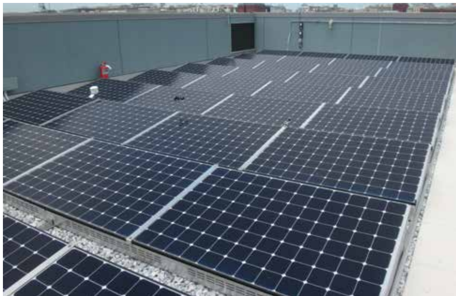
Figure 1. Example rooftop PV arrays on racks.
