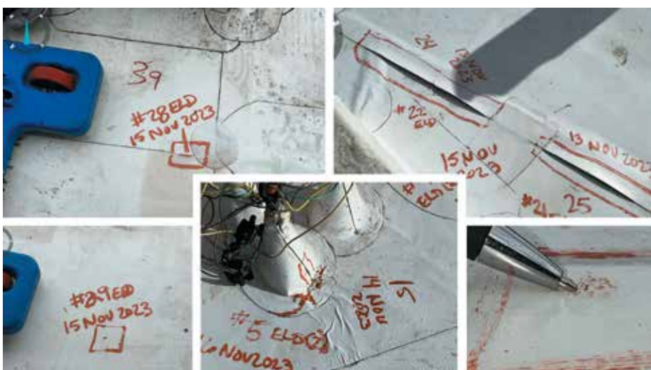
Figure 10. Examples of seam voids and punctures found at office building in California.
