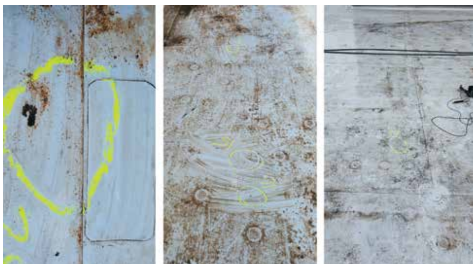
Figure 12. Examples of breaches and seam voids located at Department of Transportation in Texas.
