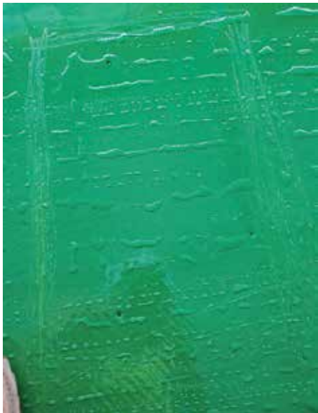
Figure 5. Examples of pinholes located at light rail station.
