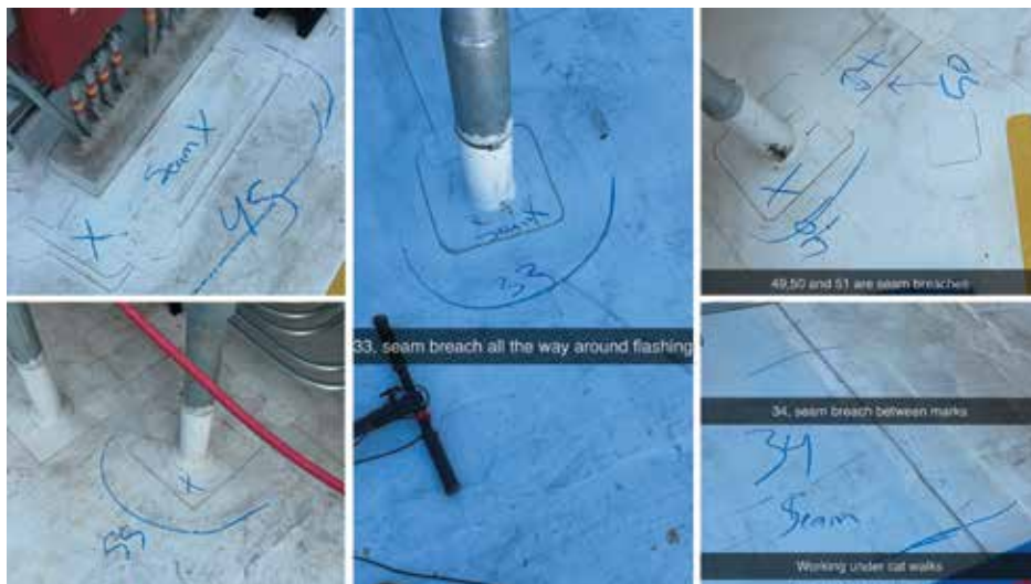
Figure 11. Examples of numerous seam voids at office towers in Washington.
