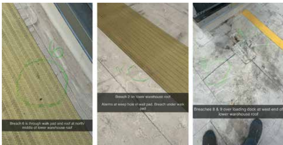
Figure 8. Examples of breaches found on one of the seven food manufacturing plants.
