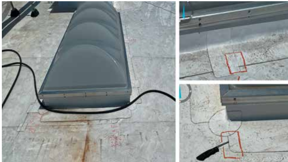
Figure 6. Examples of breaches found during forensic electronic leak detection testing at lab space in California.
