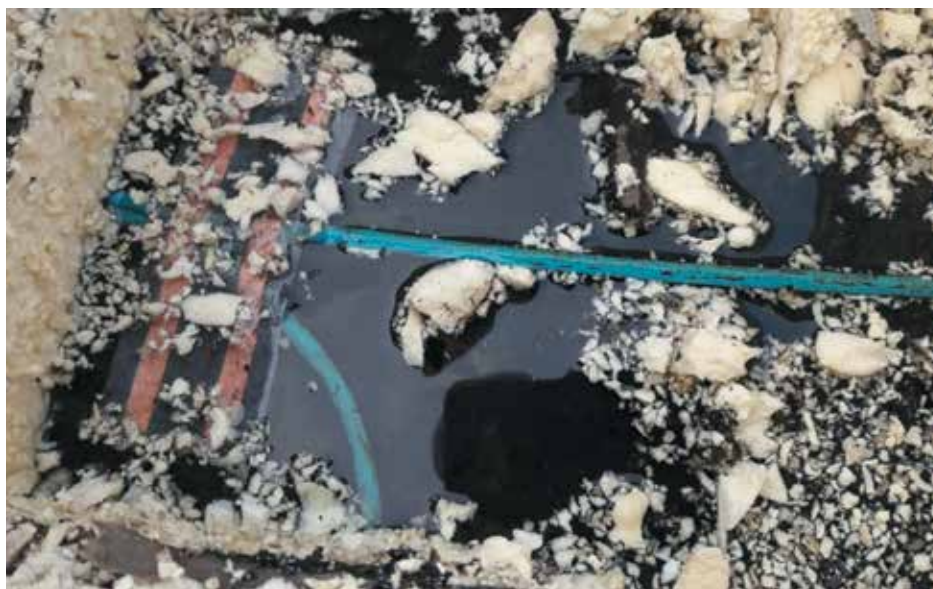
Figure 13. Standing water on moisture detection sensors at apartment building in Oregon.
