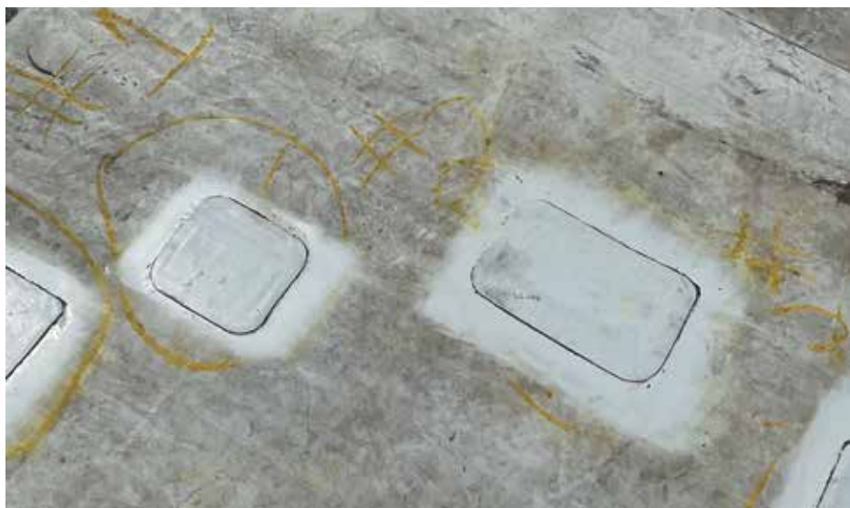
Figure 16. Breaches located, repaired, and retested at health care complex in Iowa.
