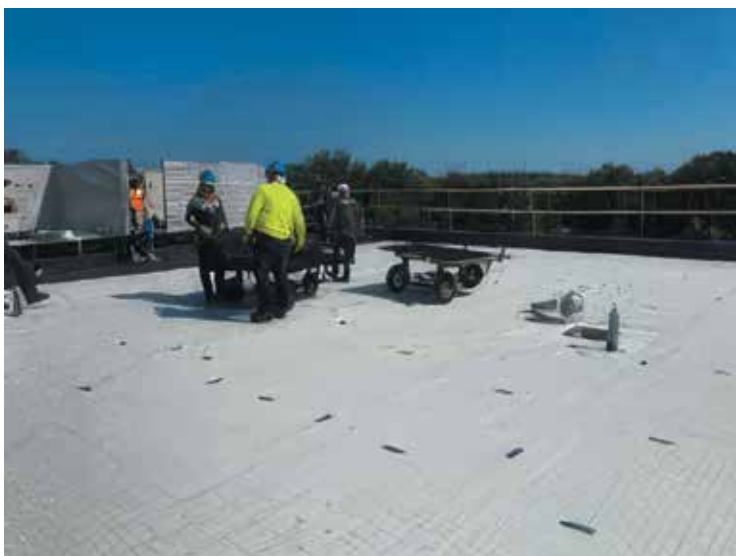
Figure 13. Roof assembly installation in progress.
