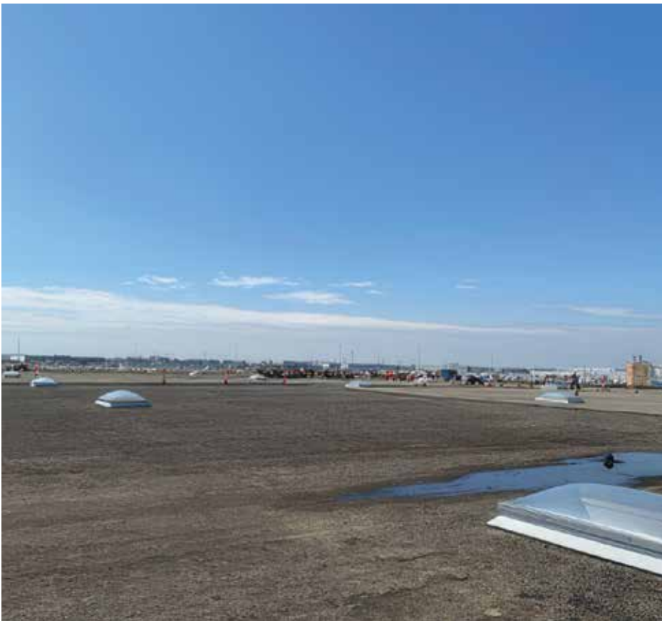
Figure 1. Existing industrial building built-up roof system.
