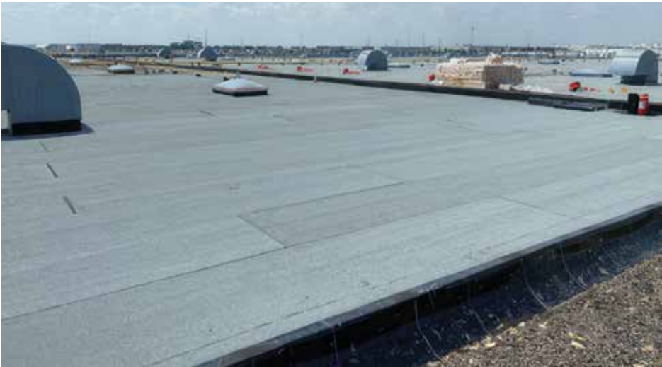
Figure 3. New roof re-cover system installed.
