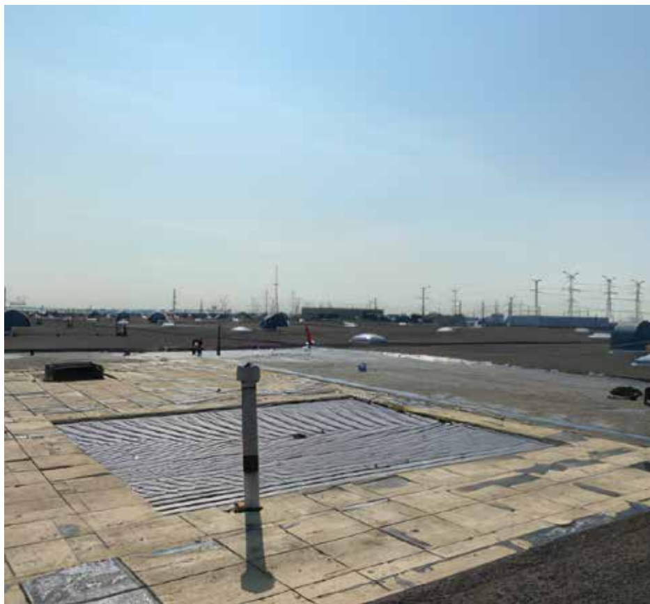
Figure 2. Existing built-up roof membrane removed and localized “wet” insulation being replaced.
